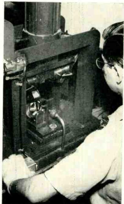
Pressing 90-degree yoke coils to shape
