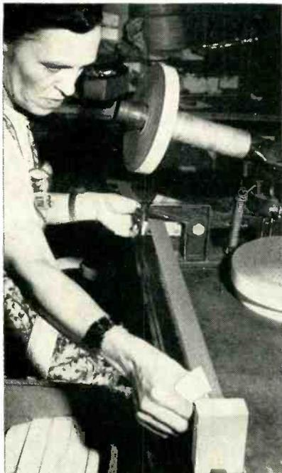
Setup for cutting picture-tube cushioning bands
