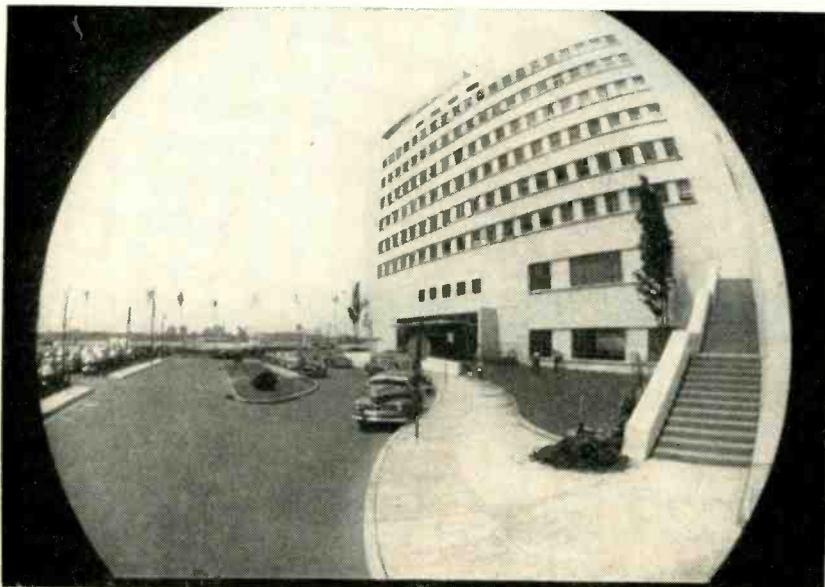
Wide-angle lens giving 142-degree field of view, as used at the Navy's Special Devices Center, Sands Point, N. Y. in a gunnery trainer. A television system using this wide-angle lens and a spherical-screen projection receiver to provide three-dimensional television is presently under development at RCA
