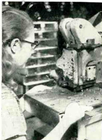
Beginning operators use template with ground riveter, but soon memorize locations of holes for ground pins
