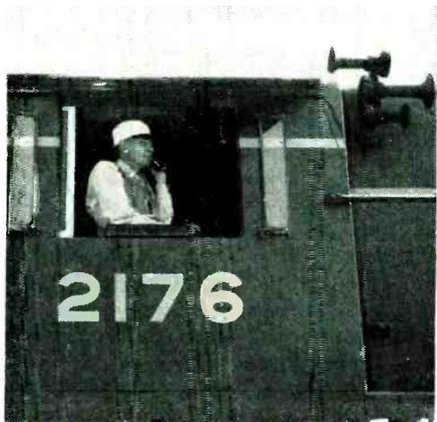
Maintaining freight-yard communications; vhf radio in switch engine features fail-safe operation. Talk-back loudspeakers keep yard workmen in touch
