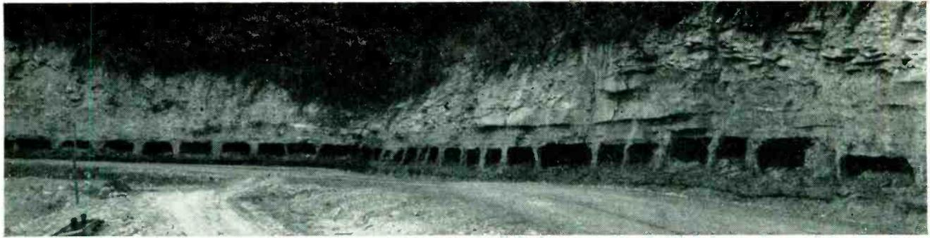
Appearance of hillside after coal vein has been mined by machine. Three-foot ribs are left between 116-inch-wide cuts to hold up hill. In present operation, holes go in only 690 feet because additional conveyors are not yet available
