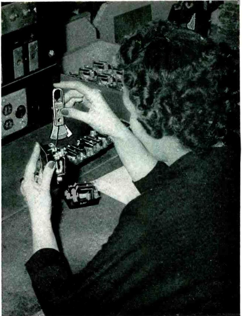
**CONTACT PRESSURE OF EVERY RELAY** is measured on a gram gauge in Ward Leonard's Mount Vernon plant.
