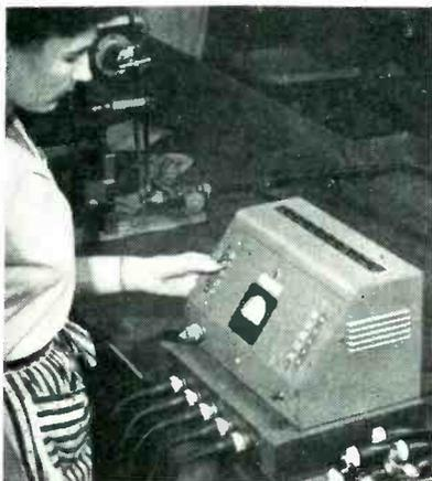
Improved version of high-voltage test set, having ten circuit-switching buttons and hence less flexibility
