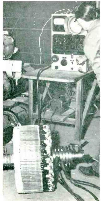
Checking windings with surge comparison tester. Similar setup is used for magnetic amplifiers
