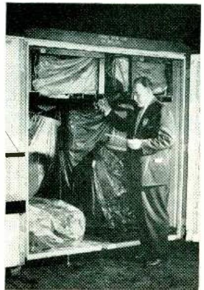
Appearance of Transportainer after all parts have been put in. When doors are closed and locked, equipment is protected just about as well as if in a safety-deposit vault. Parts are loaded in such a way that they can be removed in the correct numerical sequence for quick and easy assembly
