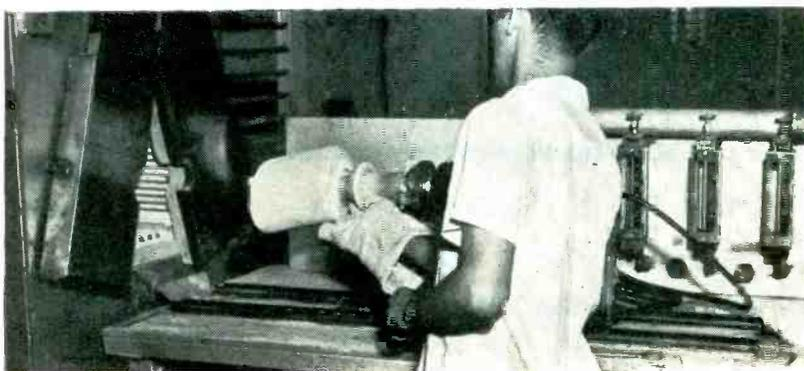
Removing ceramic container filled with resistor blanks, after coating with carbon in electric oven at left. A chain drive wobbles the container while inside the oven to give tumbling action
