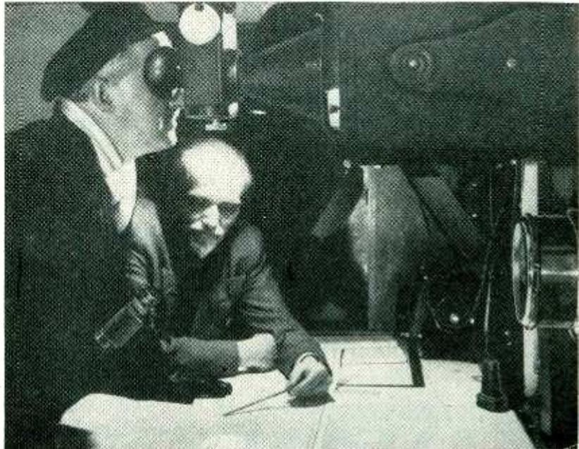
Identification of light blobs on a radar screen, indicating objects surrounding a ship, is often difficult for a navigator. A British invention makes it possible to superimpose the radar display upon a standard chart of the area. The chart comparison unit, which is attached to the radar indicator, also projects an arrow upon the chart below to show the navigator his position and heading
