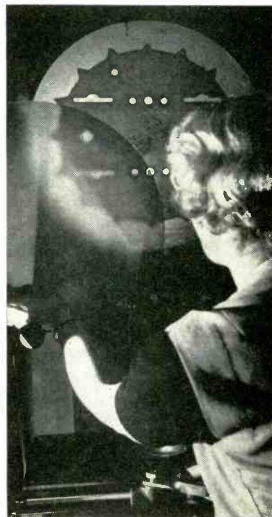
**Inspecting Tube Micacs with Optical Comparator**
