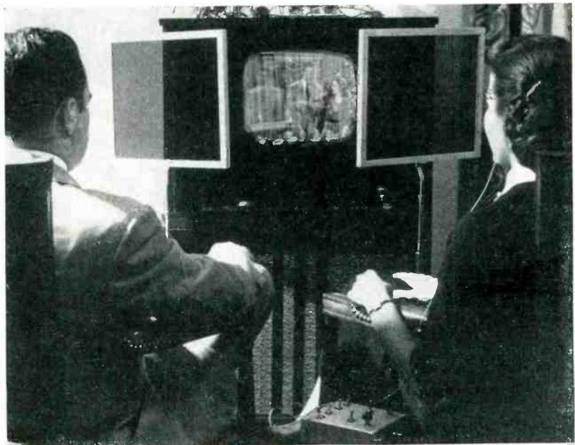
TELEVISION receiver with two superimposed images that can be separated by polaroid glasses is shown by DuMont as . . .
