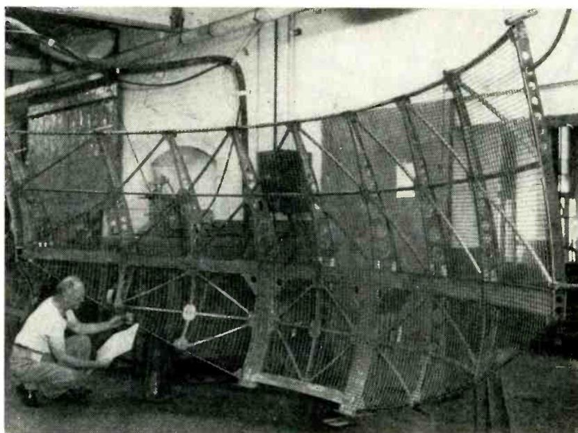
RADAR scanning screens for naval vessels are mounted high in the ship's superstructure. This imposes severe requirements for light weight, yet demands great strength to resist the winds, vibrations and pitching and tossing movements that occur in this high and exposed position. Also, though large, these
