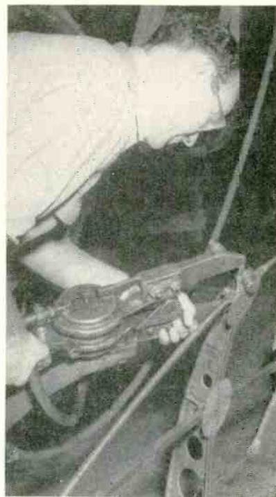
Final joining of half-inch tube members to the radar screen frame is accomplished by shot-welding the tacked joints. Lower assembly of the screen skeleton has been removed from wood shaping form and is now ready to be joined to upper assembly
