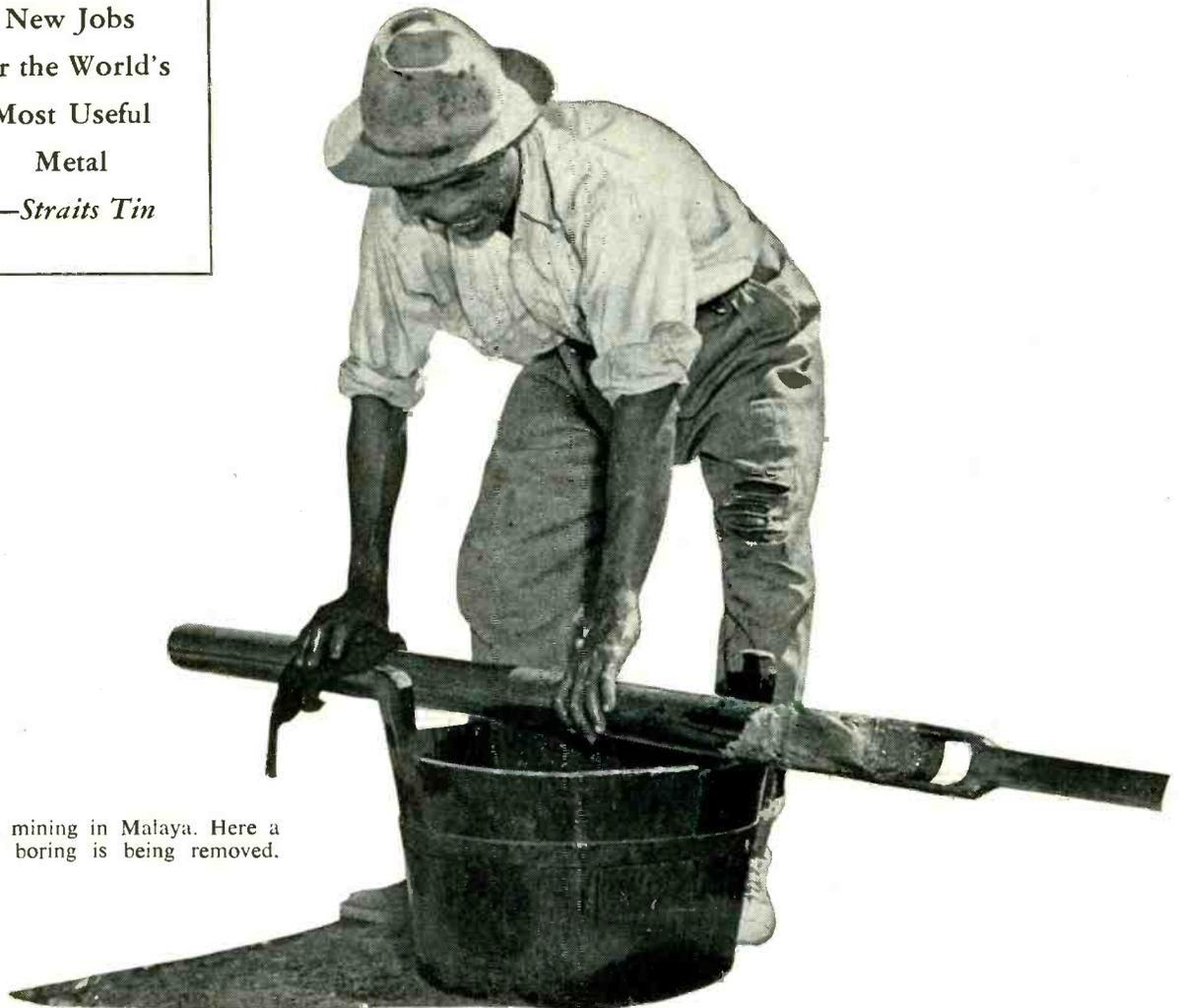
Tin mining in Malaya. Here a test boring is being removed.
