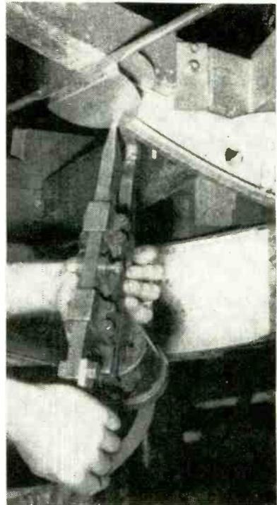
Using electric hand welding machine for welding preshaped tubing to stainless steel joint flanges which in turn are shot-welded to the vertical ribs of the radar screen. Welder is supported from ceiling on track carriage. Assembly is done on shaped wood forms having positioned brackets.
