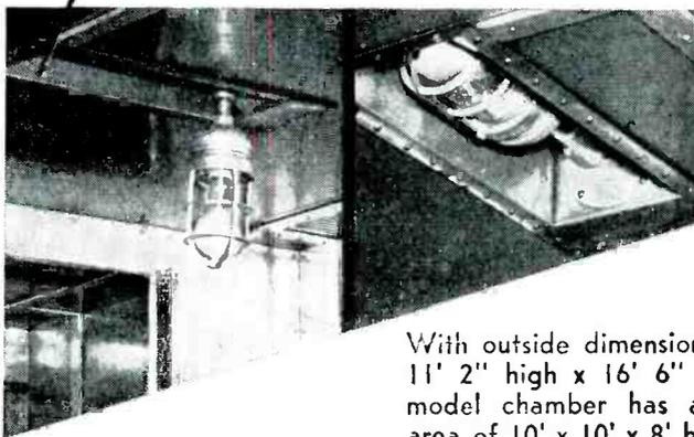
With outside dimensions of 13' 2" wide x 11' 2" high x 16' 6" long, this standard model chamber has an interior working area of 10' x 10' x 8' high. Door is 5' wide x 8' high, its window 30" x 30", and wall window 36" x 36".
