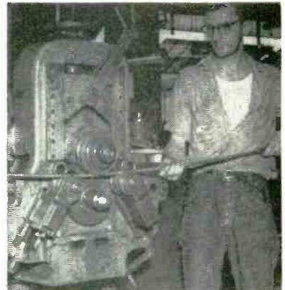
Use of three special shaping rolls to give required parabolic shape to shorter lengths of half-inch tubing. Several passes are used, with the degree of arc increased for each pass. No mandrel is needed to prevent deformation
