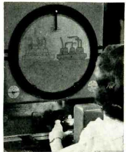
Checking length and angularity of leads in tube stems with contour projector, using screen chart having two views of stem and staging table that rotates and moves stem 90 deg for comparison with each view in turn
