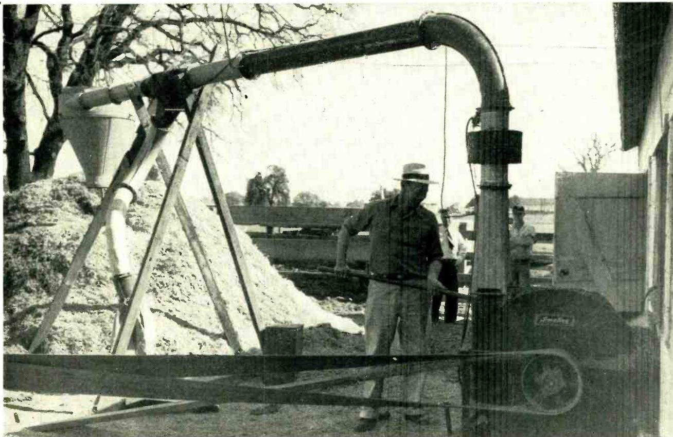
First field trial of tramp-iron remover. Total of 34 pieces of dangerous wire and nails was removed from this haystack in first pass through setup, and none on second pass
