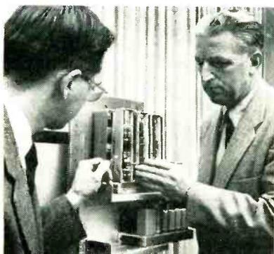
Model of a carrier-frequency telephone terminal suitable for rural lines. More than 300 transistors of the type held by man at the left are used in experimental equipment
