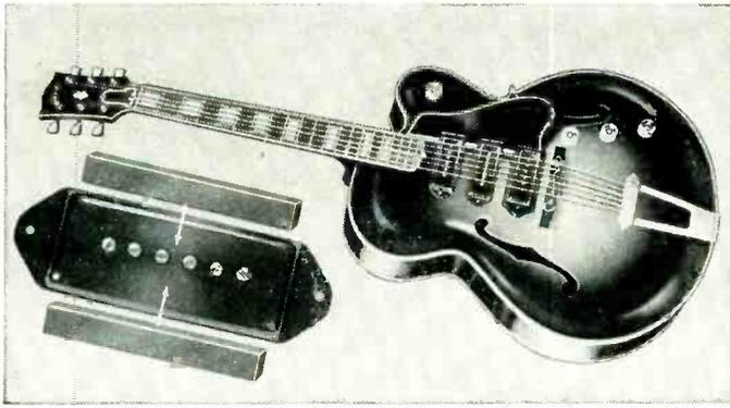
The heart of this Gibson electric guitar is the magnetic pick-up. Steel strings vibrate in the field set up by two small Carboloy permanent magnets, generating minute electrical impulses.
