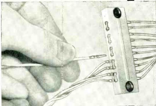
**BASIC 10 CONNECTOR TAPER-BLOK WITH DUAL CONTACTS**
