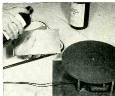
Pouring photo resist solution on copper-clad phenolic sheet
