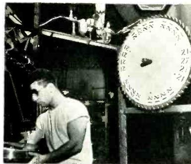
Pattern wheel at conveyor loading position, with air-actuated pawl on shelf at left rear of wheel
