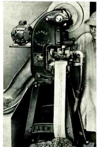
Precision gasket-punching machine in operation. Air blast from vacuum cleaner, acting through pipe at front of press, blows finished washers into hopper at rear of machine
