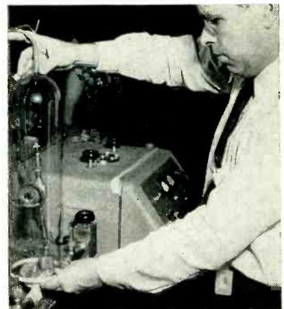
Placing helium-filled bell jar over magnetron sealed into vacuum line of mass spectrometer type of leak detector
