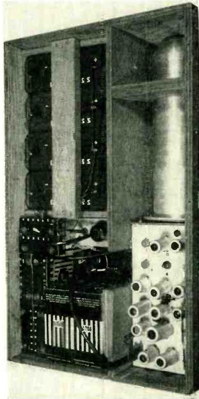
Complete gondola with radiation detector. High-voltage supply is located behind detector unit
