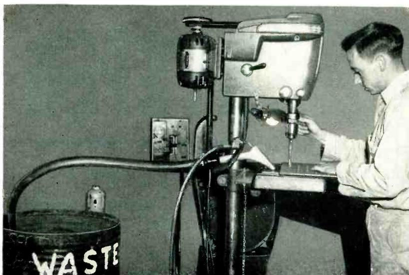
Cleaner mounted on drill press for transferring chips to waste barrel as fast as they are produced, while drilling instrument panel
