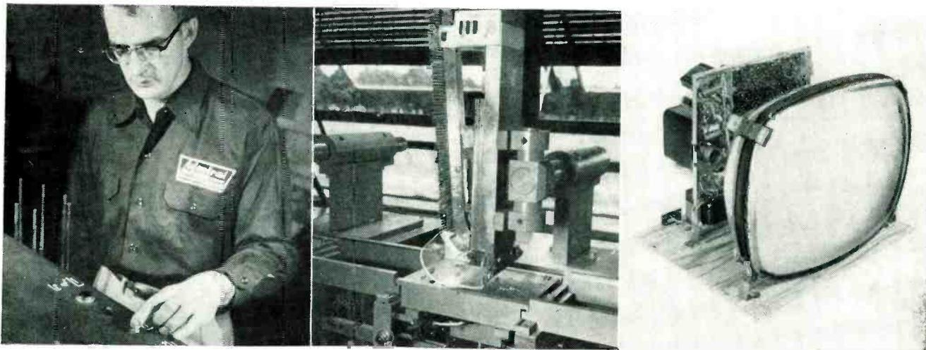
**PUSHBUTTON** starts machine that trims and bends resistor leads, inserts them in printed circuit boards and crimps them in position. Printed circuit assembly comprises nearly 50 percent of completed vertical tv chassis wiring as . . .
