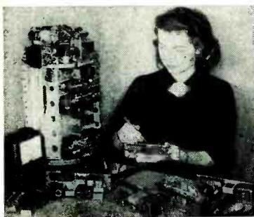
**C**OLOR is used to identify plug-in chassis that form part of airborne radar navigation equipment designed by General Precision Laboratory, Inc. Features of the radar include ability to function under a wide range of environmental conditions and use of standard tubes having normal tolerances.
