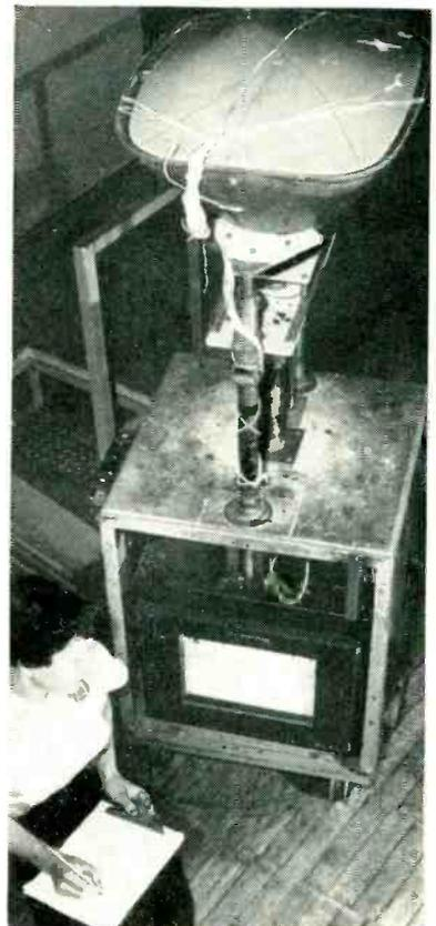
Recorder cart with picture tube is taken out of production line after trip through oven, for analysis of recorded data
