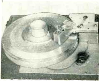
Four-channel magnetic record-playback head and turntable
