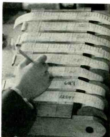
Strip charts used for recording numbers of rejects in each batch of 100 tubes of a given type. Noise, electrical and mechanical defects are listed separately in a vertical row of three boxes
