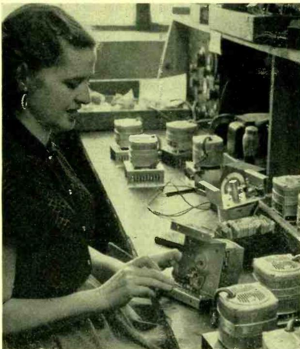
Inspecting instrument-motor chassis. This device forms part of a supervisory control system by which heavy equipment such as oil-refinery pumps can be regulated by signals from a central location
