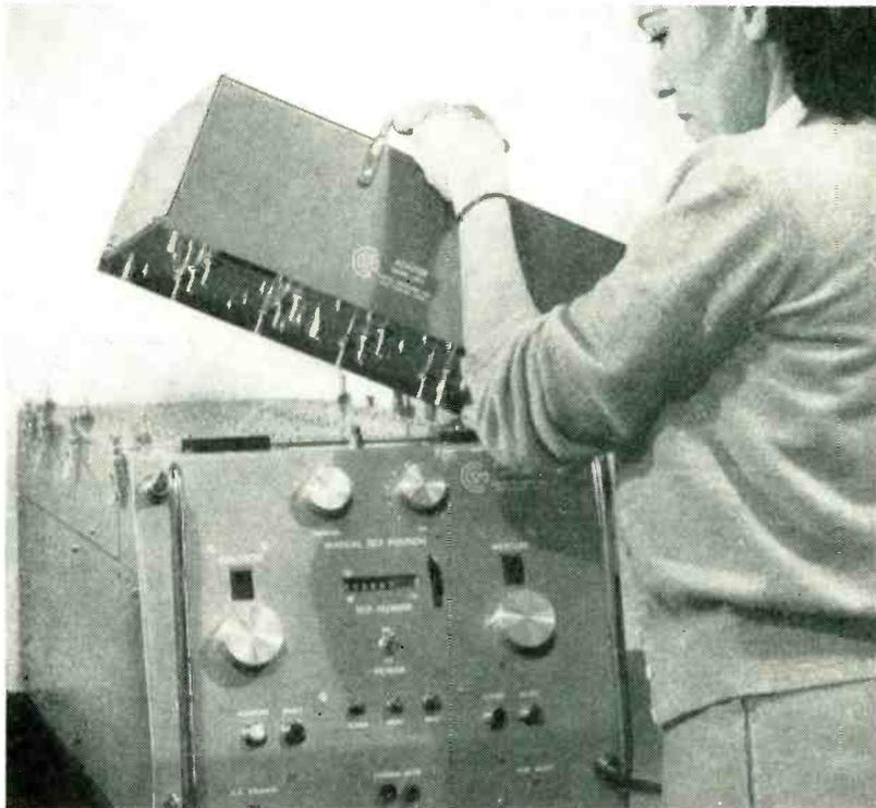
Adapter unit (at top) contains programming and selector switches
