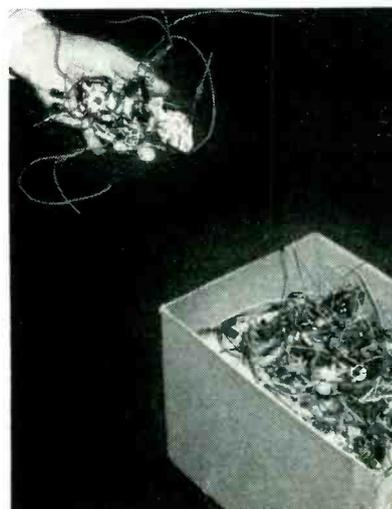
With jigs removed, subassemblies are stored in cardboard box until needed in final chassis
