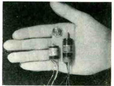
motor illustrated has the following performance characteristics: no load speed, 6,500 rpm; stall torque, 0.1 in. oz; power input per phase, 1.5 w; voltage input per phase, 18 v; and weight, 1.2 oz.
