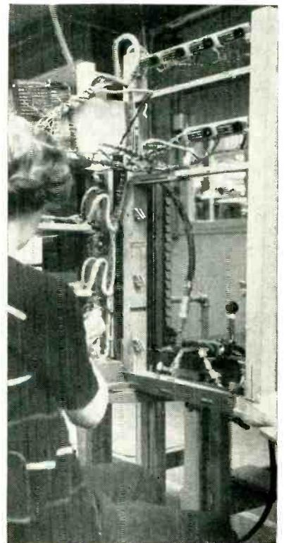
Completing assembly at bench height, using cleats and brackets on uprights to hold wiring harness and attached parts
