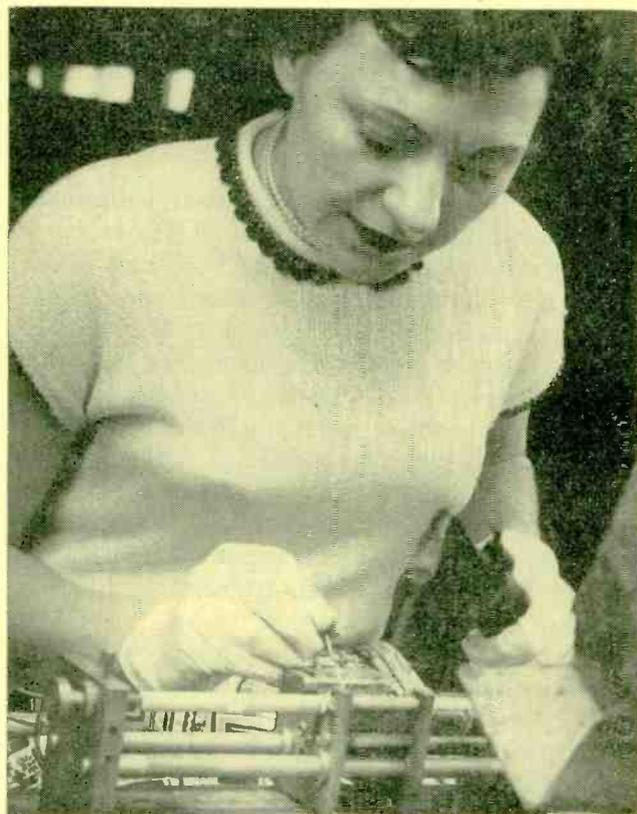
FIG. 7—Use of a torch in soldering operation. Operator is assembling variable air-dielectric capacitors
