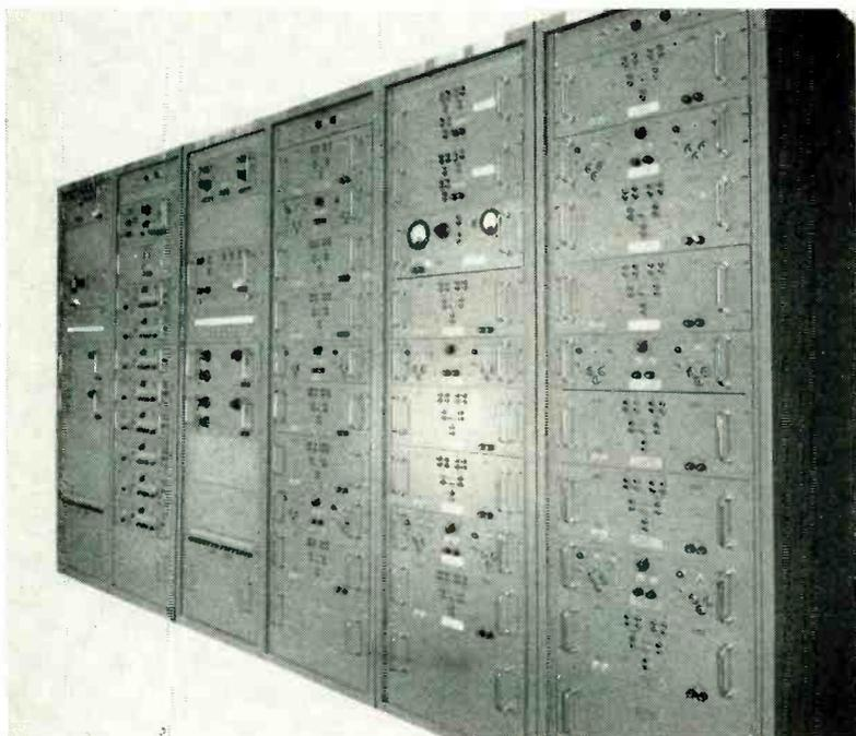
FIG. 1—Complete carrier-telegraph terminal. Two transmitting cabinets are at left. Four others are for receiving circuits
