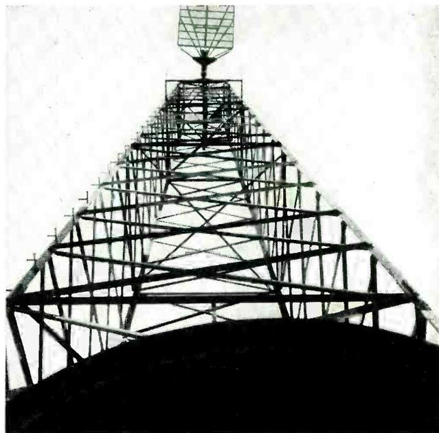
Supervisory control panel illustrates how microwave operates an unattended remote pipeline booster station. Passive reflector mounted on steel tower is becoming symbolic of a new communications age
