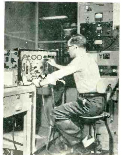
New Signal Corps radio transmitter AN/TRC-24 undergoes Western Electric tests in shielded room. Equipment, to which engineer is making adjustments (right hand on knob) is part of multi-channel communication relay system that links points up to 30 miles apart by radio
