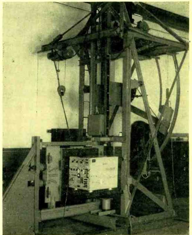
Mechanical testing. Console of radar fire control equipment is shown undergoing vibration test on shake table, left. Shock tester, right, delivers either horizontal impact shocks, by hammer, or vertical shocks by dropping test platform
