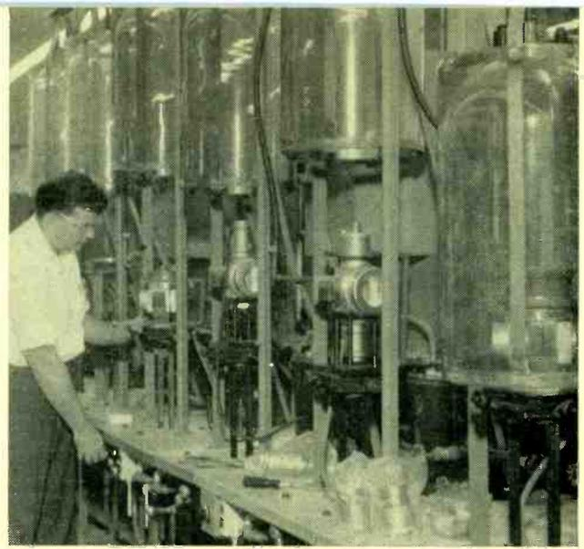
FIG. 6—Joining magnetron cathode structures by high-frequency induction brazing. Bell jars maintain controlled atmosphere 90 percent nitrogen and 10 percent hydrogen to prevent oxidation
