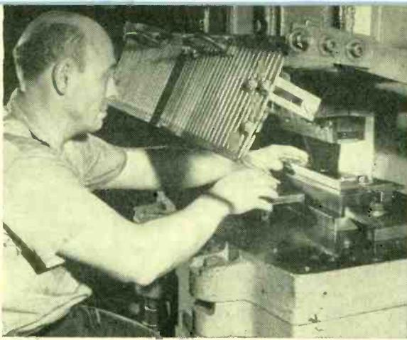
**DESIGNING THE CHASSIS** involves selecting materials, laying out the work and specifying the finish. Operator is punching out subassembly chassis with a 75-ton geared press
