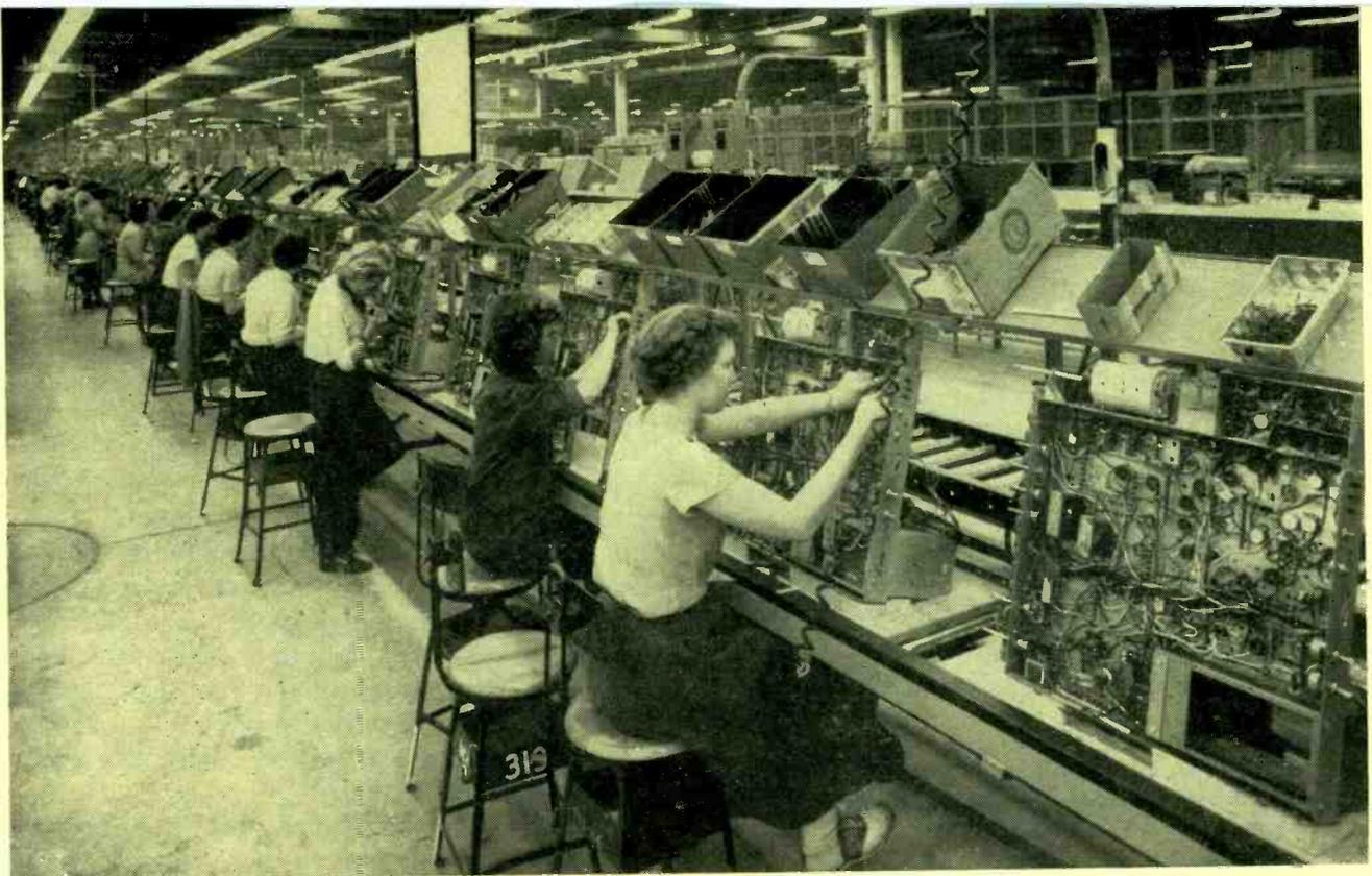
Wiring and soldering operations, often performed along a moving belt like the one shown, may represent 30 to 40 percent of direct labor cost in manufacturing electronic equipment
