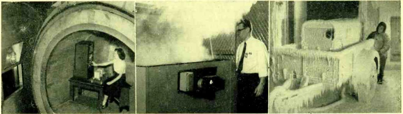
Environmental testing. Equipment at left is readied for test in Signal Corps' stratosphere chamber. Center photo shows chamber for 50-hour salt-spray test. Resistance to ice and snow is determined by testing equipment in cold room, right
