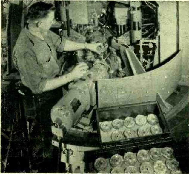
FIG. 3—Multispindle automatic machine drills, reams, chamfers, faces and taps 750 telephone-dial frames per hour. A 12-position die is used. Tolerance on center hole is  $+0.003$  in.,  $-0.000$
