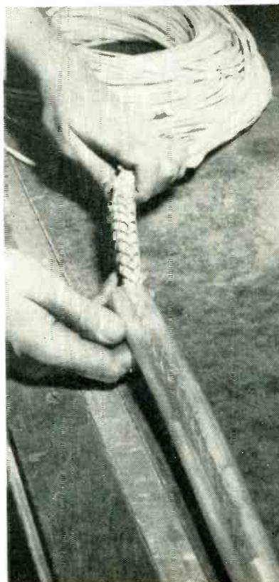
Guiding cable grip and conductors into tubing as operator at other end of tubing winds up cable on drum
