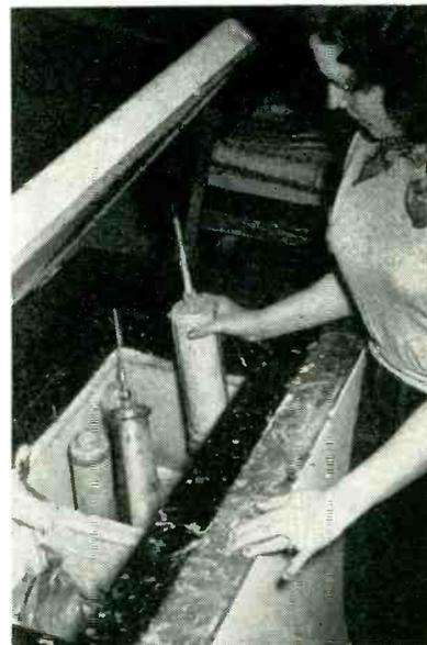
Method of storing dispensers in deep freezer. Some compound is placed in plastic bag as at left; this can be taken to an aircraft for filling plugs that are already in position. This is done by cutting off a tiny corner of the bag and then squeezing the bag to force out the compound
