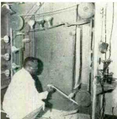
Tape spray chamber, with spray gun at right. Infrared lamps dry coating
