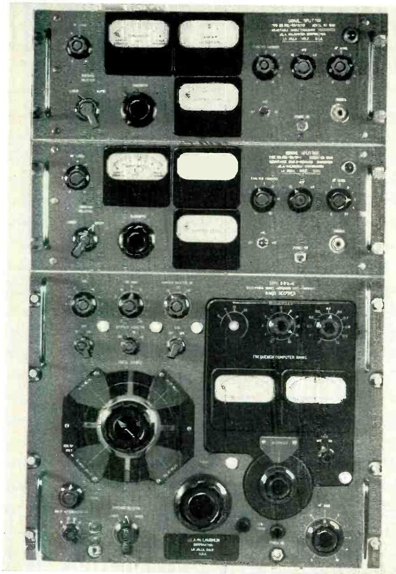
Selectable single-sideband dual-diversity receiver with single-sideband converters (top) for electronic bandwidth control
