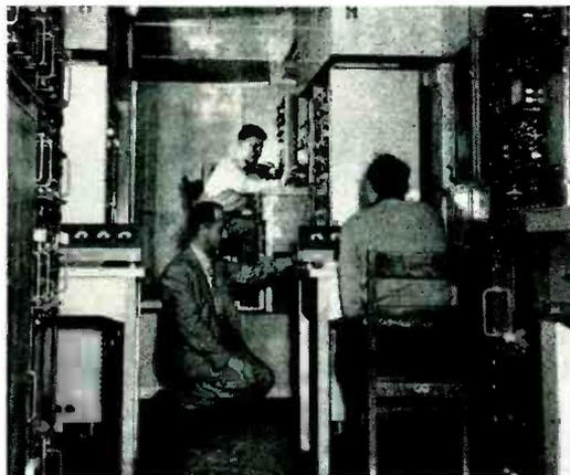
Inside this mobile ground station, test flights of the Avro Canada CF-100, RCAF all-weather interceptor for continental defense, are "seen" and "heard" with Ampex magnetic tape recorders.
