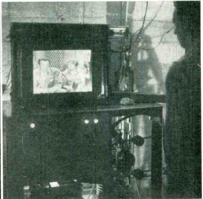
**POSITIONING** cathode-ray-tube electron gun at side instead of rear of glass envelope reduces tube depth to approximately 3 inches. Laboratory model of black-and-white version of tube, shown in operation, helps . . .
