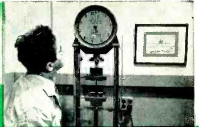
One reason UTC transformers can carry a strong materials workmanship performance guarantee is that all incoming materials are thoroughly tested against specs before they are accepted and used. Here, tensile strength of insulation is being checked.
