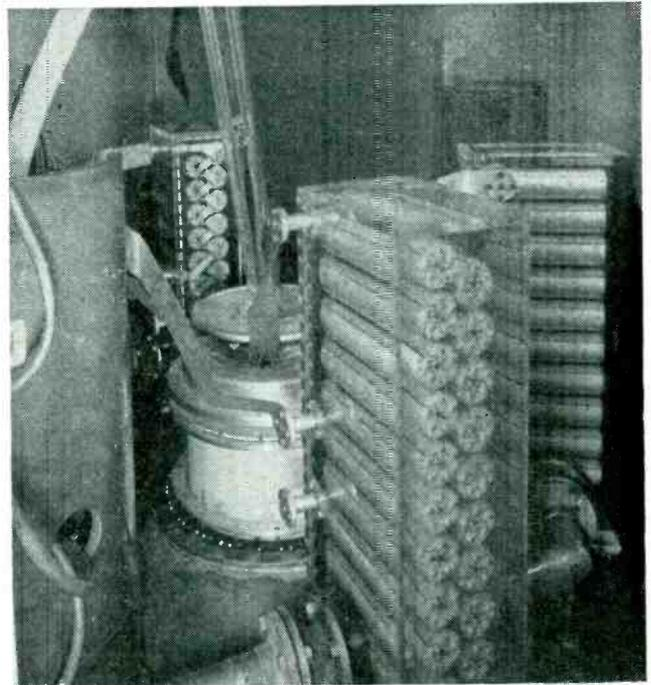
Inside r-f house, north tank. Cylindrical unit is final amplifier, surrounded by inductor boxes
