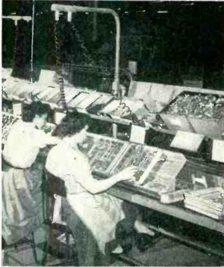
Start of assembly line for i-f strips, showing operator loading strips into four-strip rack
