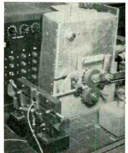
Artos drive and chopper with protective housing removed. Pushbutton in left foreground clears counter and actuates chopper as required after threading in new wire
