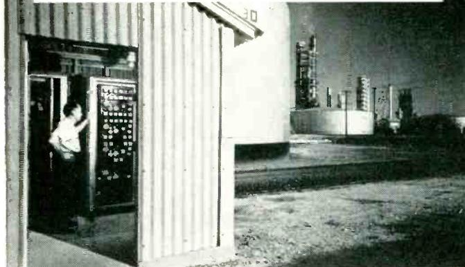
**A Second Benefit:** These pumps at the tank site are controlled instantly and accurately from the loading terminal.
