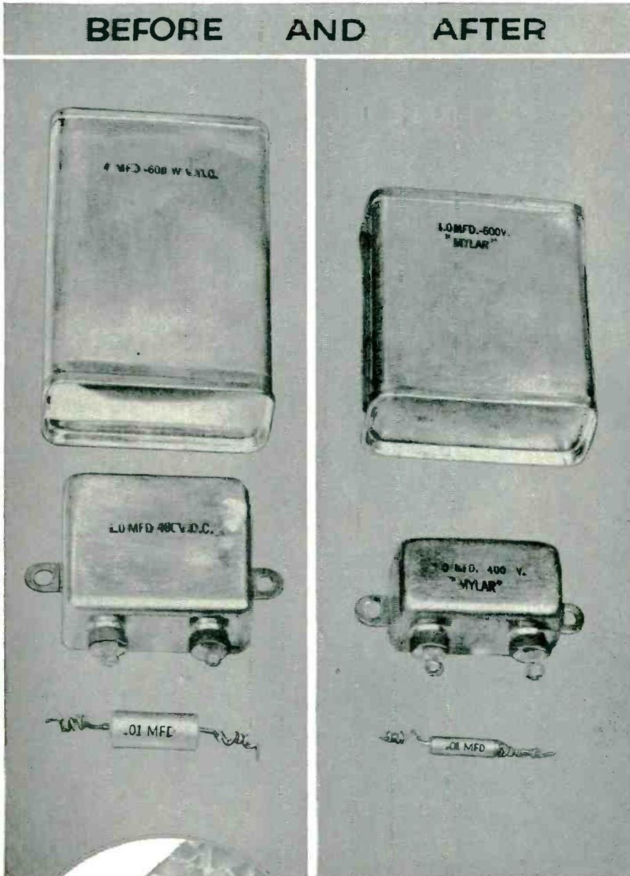
Used as dielectric, new Du Pont "Mylar" makes possible significant size reduction in capacitors.
