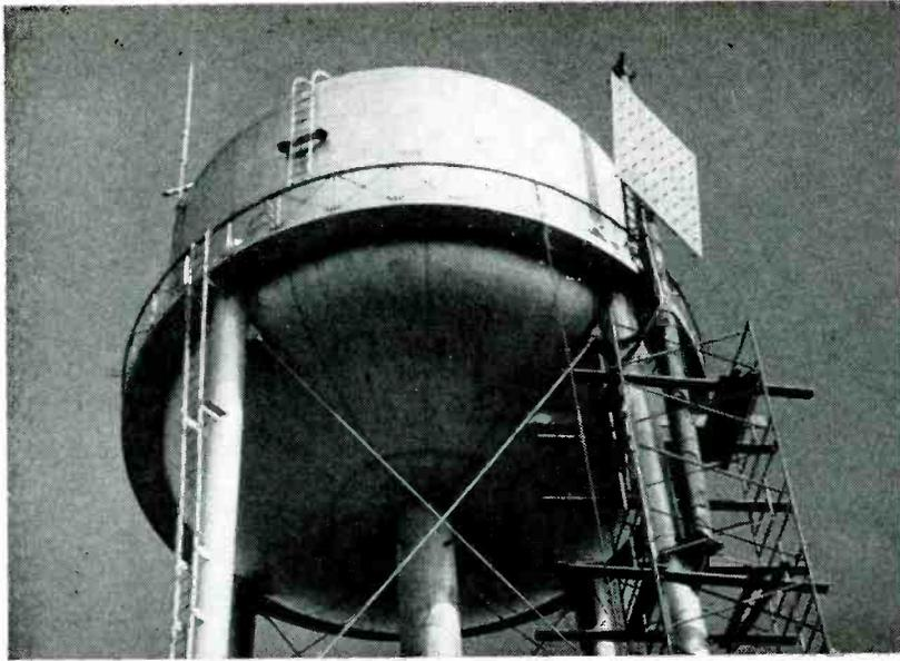
Billboard type of receiving antenna is mounted on nearby water tank and connected with the amplifier through coaxial cable
