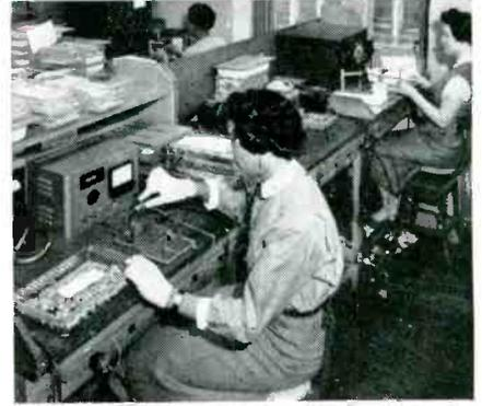
Each unit, from start to finish, is checked at least 5 times for voltage and capacitance before being shipped. In this step, capacitors are tested at DC voltages at least 200% of rated voltage at 25°C.
