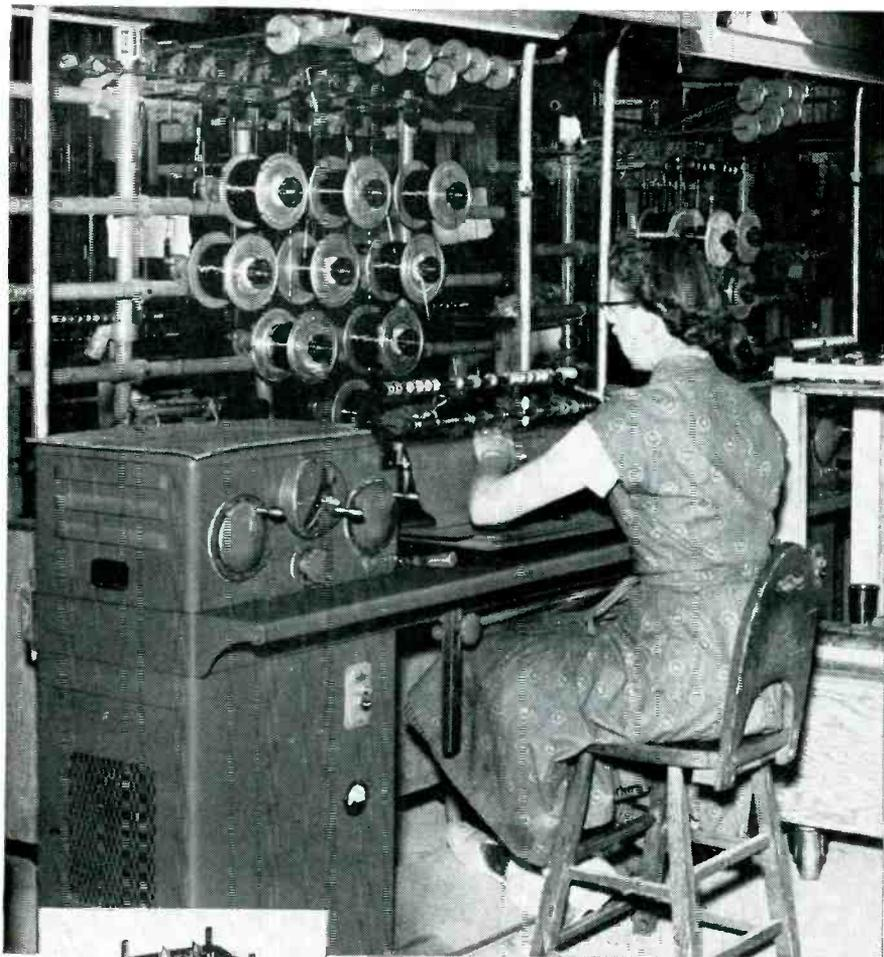
At the Freed Transformer Company, well known manufacturers of electronics components, Leesona No. 108 Hand-Feed Coil Winders have replaced obsolete winding equipment. Here's what the president of Freed reports about the new installation:
