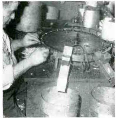
Automatic shorts tester for selenium rectifier cells. Good cells are blown into container at right of operator. Turntable rotates clockwise
