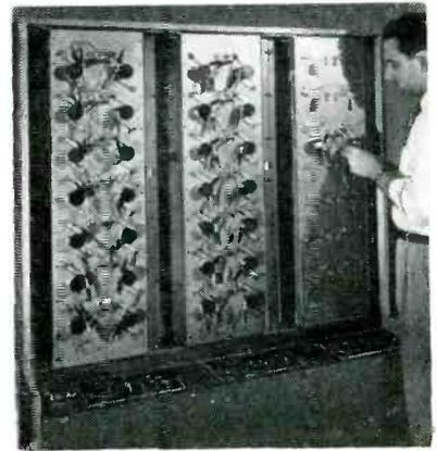
Three-bay, six-door unit for testing 84 units at a time. Metal strips locked in position by wing nuts hold potentiometers in position on doors
