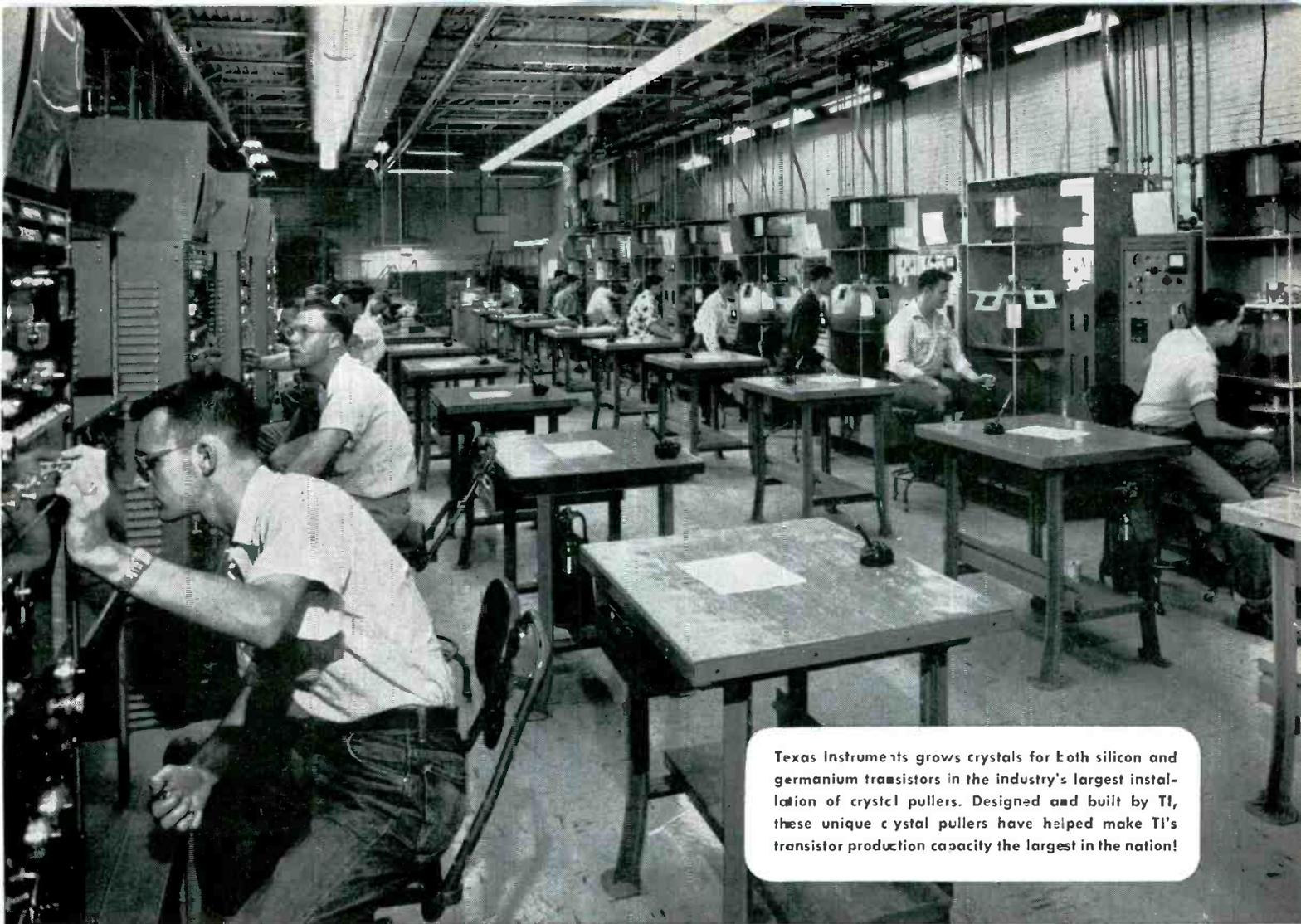
Texas Instruments grows crystals for both silicon and germanium transistors in the industry's largest installation of crystal pullers. Designed and built by TI, these unique crystal pullers have helped make TI's transistor production capacity the largest in the nation!
