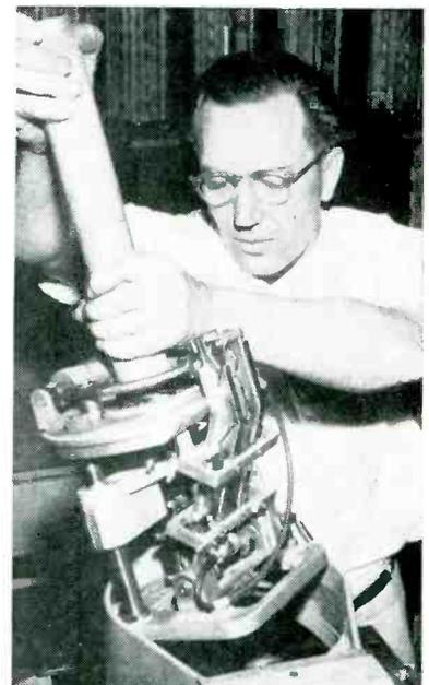
Removing insertion head
