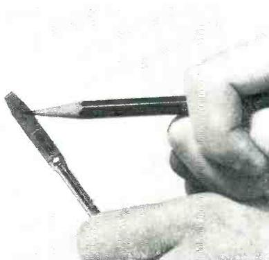
**RAPID HEAT TRANSFER** is achieved by locating the heater directly in the ironclad-copper tip. Result—the G-E Midget iron's heat efficiency is 90%.
