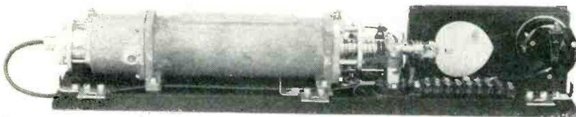
Heart-shaped cam actuates plunger in coaxial oscillator to change frequency
