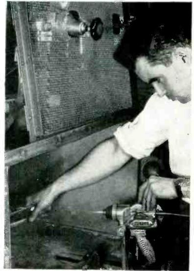
Spraying resistance card with molten metal to form end connections, using combination mask and holding fixture
