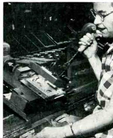
Bringing up lever to press down newly inserted components preparatory to cutting and clinching
