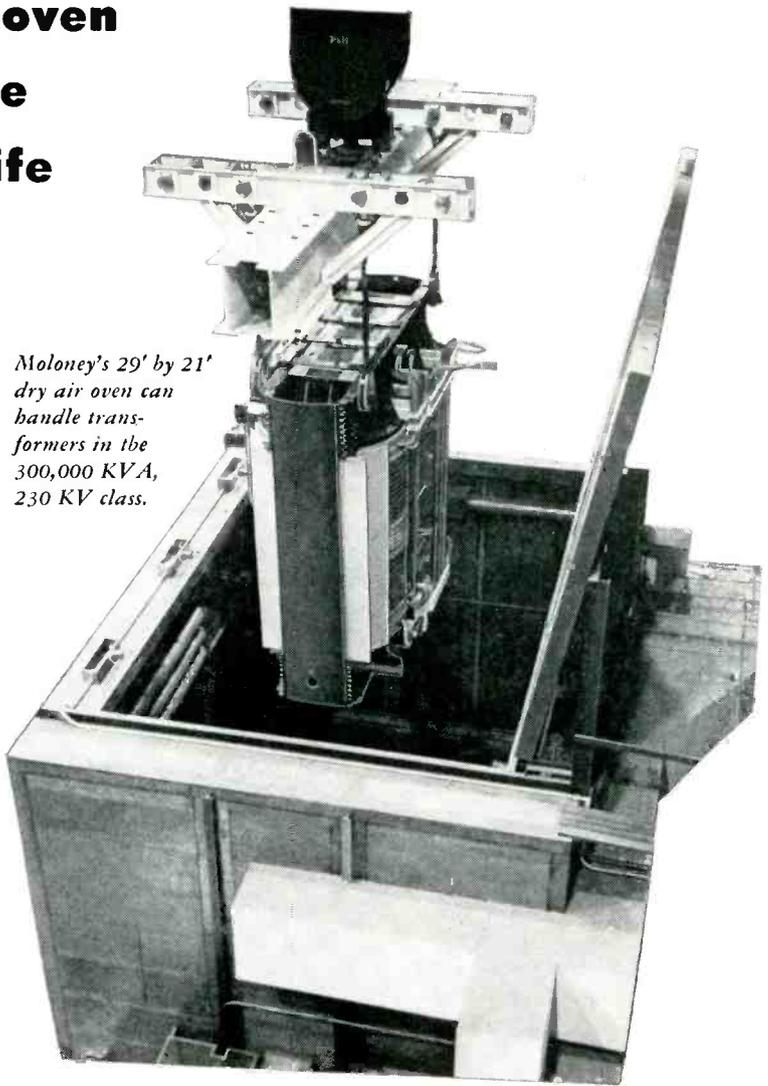
*Moloney's 29' by 21' dry air oven can handle transformers in the 300,000 KVA, 230 KV class.*
