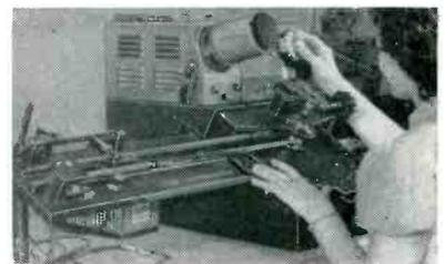
Linearity checking setup, with resistance card on fixture in front of B battery. Contact arm running over card is moved by stainless steel belt going over shaft of master potentiometer in front of operator
