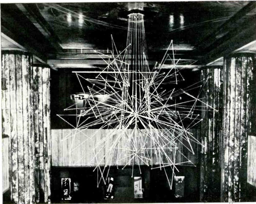
**What carries the current** in the wireless chandelier of New York City's Barbizon-Plaza Hotel? The fixture is constructed of gleaming Inco Nickel tubing in an intricate pattern — and the tubing carries the current! Nickel tubing is light and rigid, too — so the chandelier can be slowly rotated from above. The chandelier was designed by Richard Kelly and fabricated by Edison Price — both of New York City.
