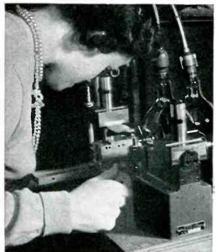
FIG. 6—Optical setup for checking concentricity of etched holes in germanium pellet. Required precision of alignment increases with operating frequency of transistor. Production and inspection controls are now adequate for at least 100-mc transistors
