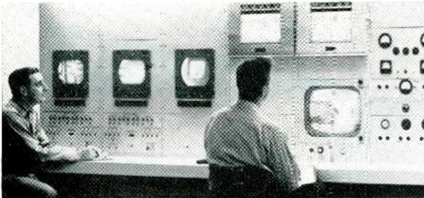
Three strategically placed RCA television cameras in the new 10-by-10 foot supersonic wind tunnel located at Lewis Flight Propulsion Laboratory, Cleveland, permit safe observation of tests. Monitors shown are installed at the tunnel control room
