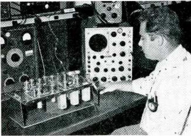
Experimental frequency shifter and demodulator undergoing test
