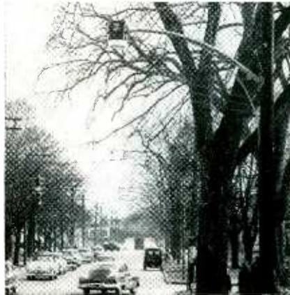
RADAR hanging from stanchion, left, detects cars approaching intersection and sends count to computer, right, that controls traffic lights when . . .
