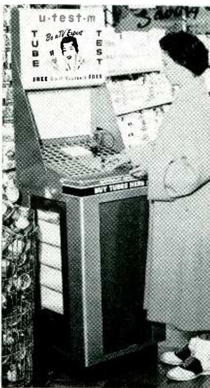
Typical grocery supermarket installation. Multiple sockets minimize control settings needed for test
