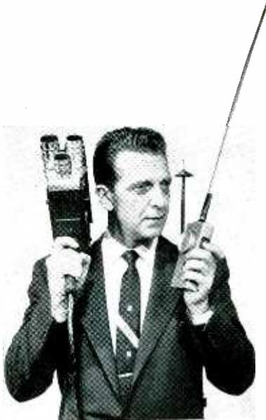
Newsman for NBC-TV's convention coverage holds experimental RCA transmitter, left, and a portable tv camera powered by a pack on his back
