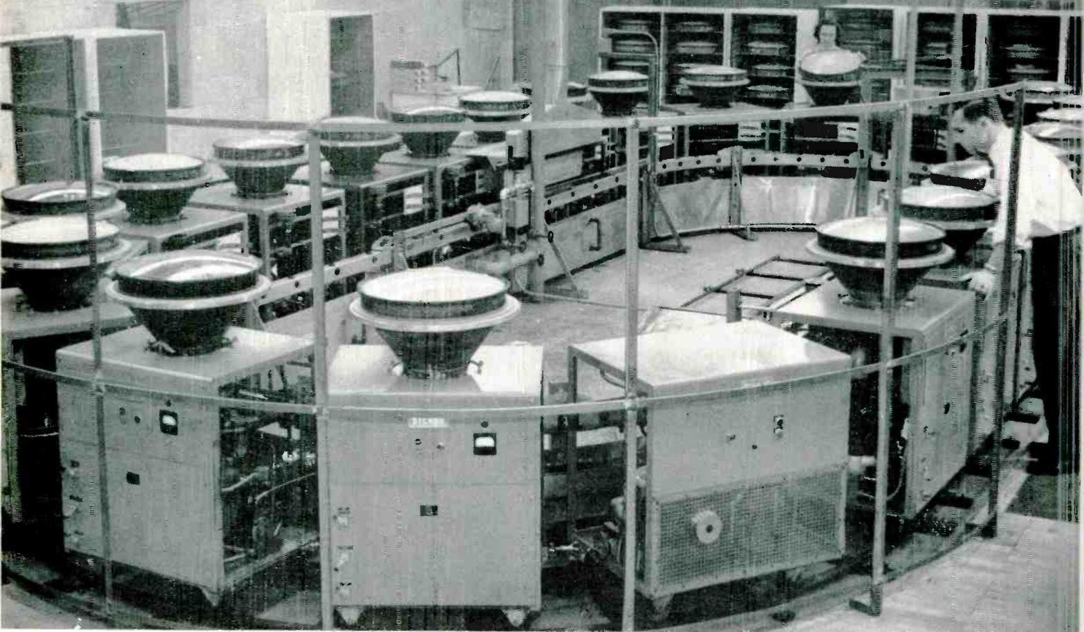
Automatic production at high output per man-hour is obtained from this complete in-line Stokes aluminizing system, used for color TV tube face plates at the RCA tube plant, Lancaster, Pa.
