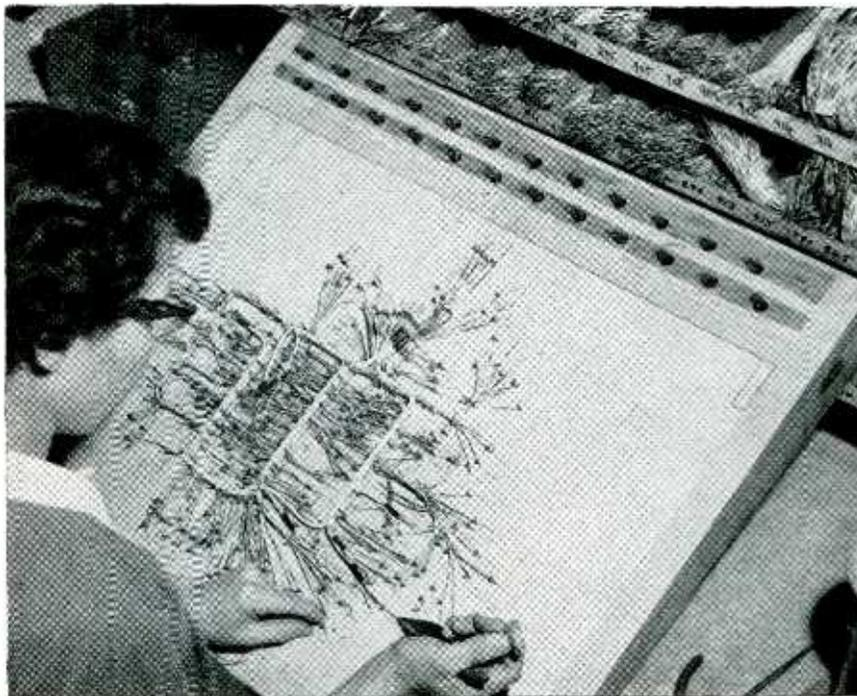
Installing wire lead on self-checking harness board. Each of 24 lamps across top of board indicates correct installation of an average of seven wires, installed in a prescribed sequence
