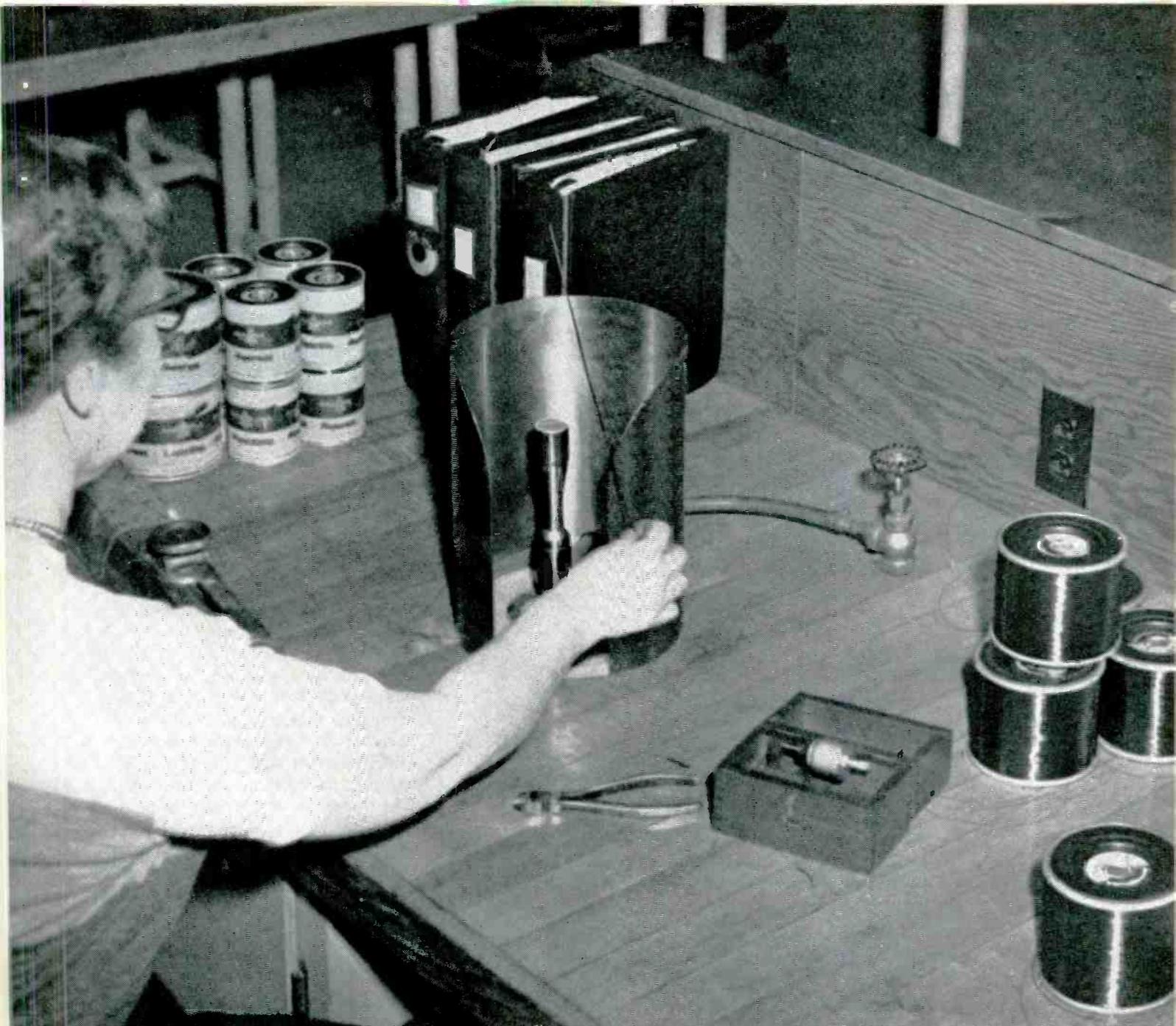
CLEANING THE INSULATION from enameled magnet wire, laboratory technician prepares to check conductor to see that it measures correctly after running through insulating machines.
