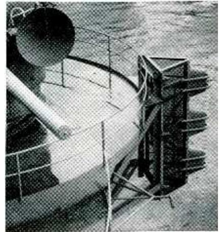
antenna, used with system developed by Federal Telecommunication Labs. Antennas for uhf communications are visible at the corners of the flight deck. Detail of similar antenna mounted on gun tub is shown at right. Eight antennas provide 360-degree cover
