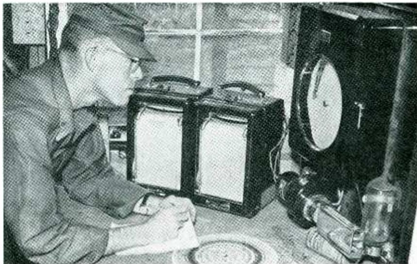
Officer checks wind direction, velocity and humidity at base of 200-foot tower. Recorder at left is connected to wind vane, the center recorder indicates velocity of an anemometer. Motor operated psychrometer and recorder are at right
