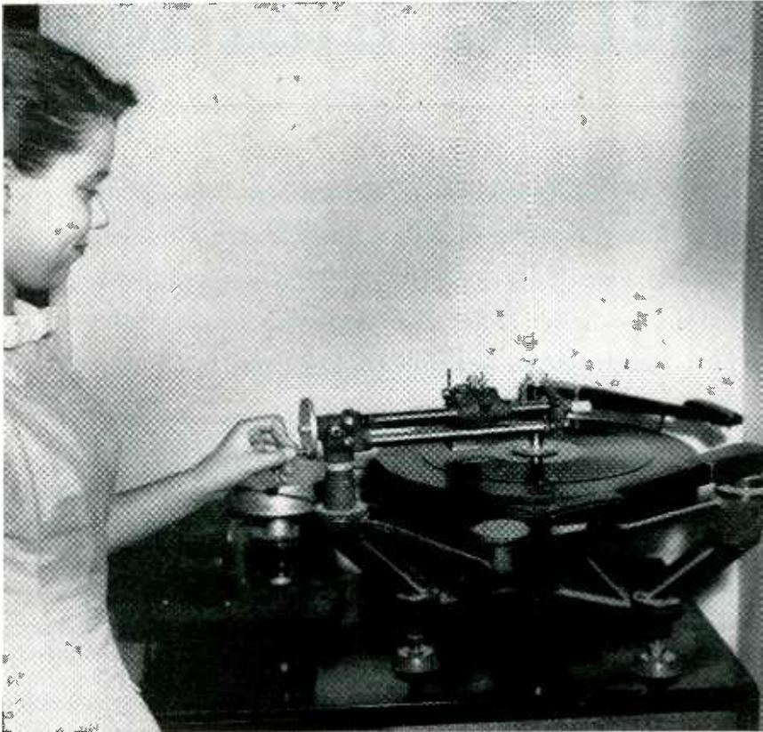
Speed of disk recorder used in tests was cut in half by using special pulley for belt
