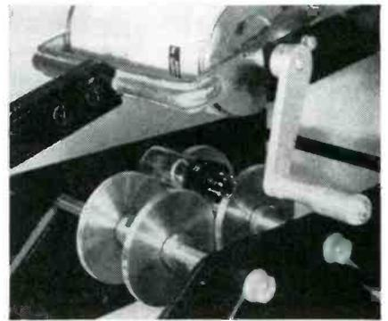
Tube to be imprinted is placed on free-turning disks, cylinder holding inked rubber type is lowered and crank is turned to place desired imprint neatly on tube base
