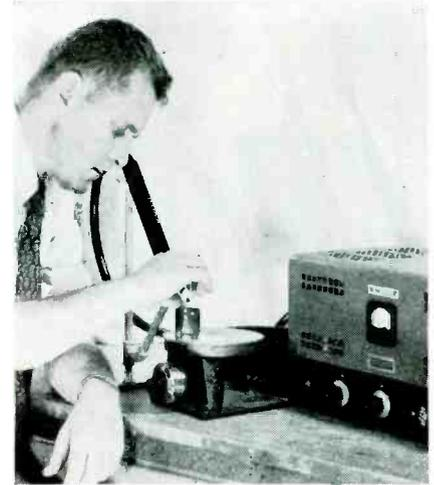
Setup for hand dipping of unstripped polyvinyl acetal enamelled wire in molten solder on hot plate, with ultrasonic unit immersed in solder
