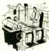
▲ At General Electric Co. — Trumbull Division — measuring operating time of circuit breakers.
