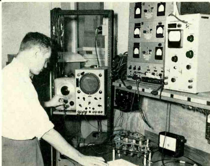
Breadboard version of electronic shutter under test. Author adjusts audio oscillator to deliver 24-cps signal to squaring amplifier at rear on bench whose 24-cps square-wave output simulates film exposure pulse. Another square-wave generator, on shelf at right, delivers 15,750 pps to simulate tv H pulses
