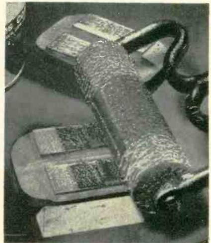
Applying cement to face of Alnico magnet
