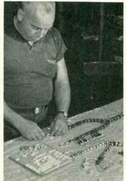
Placing identifying sleeves on leads. Adhesive-faced cardboard in front of operator serves as tote tray for sleeves
