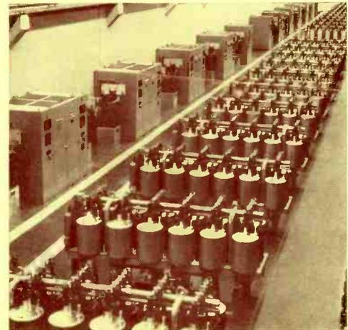
LEFT: a continuous air-tight weld of ignitron covers to tanks is formed by rotating the big tubes in motorized jigs. RIGHT: showing a large rectifier installation of G-E pumpless ignitrons. Note the clean layout, free from vacuum pumping equipment, headers, gages, and connections. Eliminating these components saves substantially in equipment, power, and maintenance costs.
