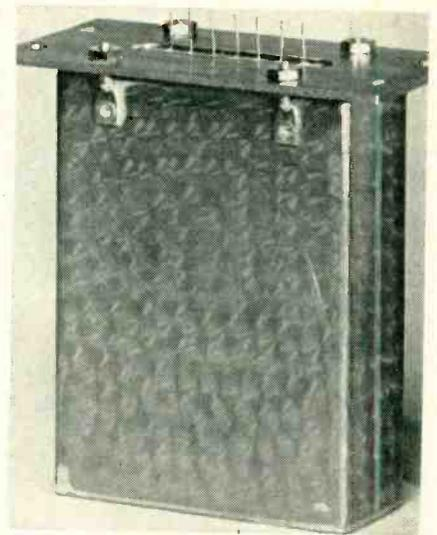
transformers using Ceroc or other ceramic-insulated copper conductors and iron cores have been successfully built and tested.
