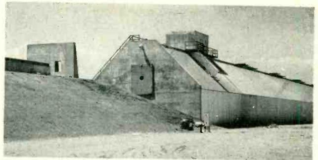
Ordnancemen load one of guns on mound outside laboratory. Projectile is fired through rectangular hole into Aeroballistics Laboratory, shown at right, in which range stations are located
