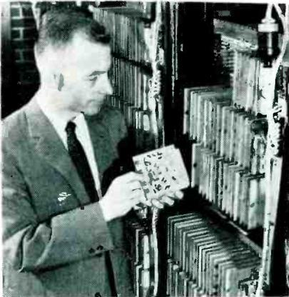
Plug-in type computer uses printed circuits, 1,500 transistors and 11,000 diodes as part of radar track-while-scan system that automatically tracks up to 72 targets in three dimensions. Developed by Westinghouse, the system presents three-dimensional information from a single-radar source
