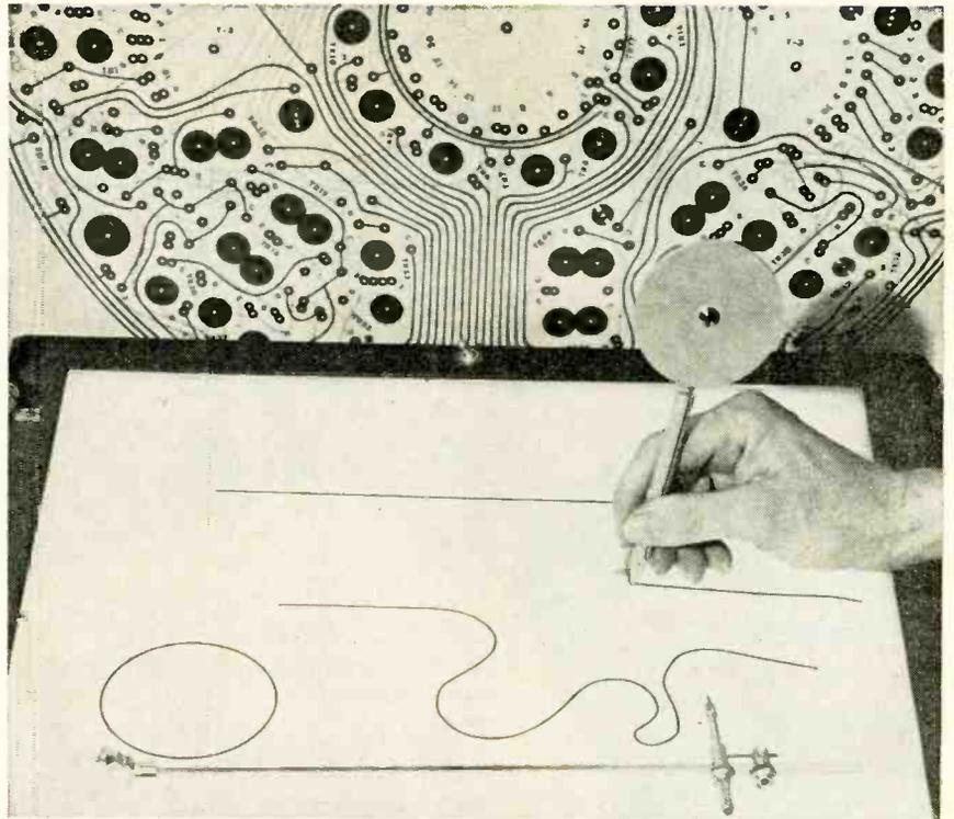
Writing with photographic tape applicator is demonstrated in front of composite layout used as guide in assembling satellite instrumentation printed circuit cards
