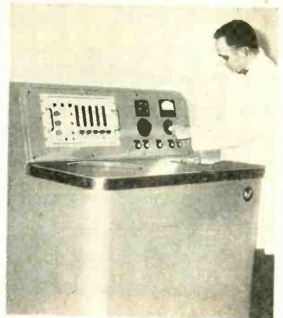
Failure-prone components are weeded-out by centrifuge tests up to 50,000 G's
