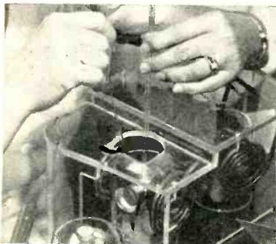
Glass seal is applied while tube is between heating coils. Tube at right is being brought to sealing temperature
