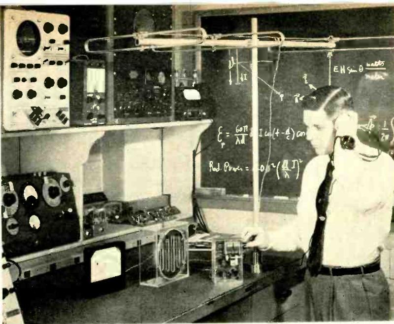
Author tunes information circuit of radiation powered transistor receiver. Operating voltage for information and audio amplifier circuits is provided solely by r-f energy extracted by and stored in power circuit
