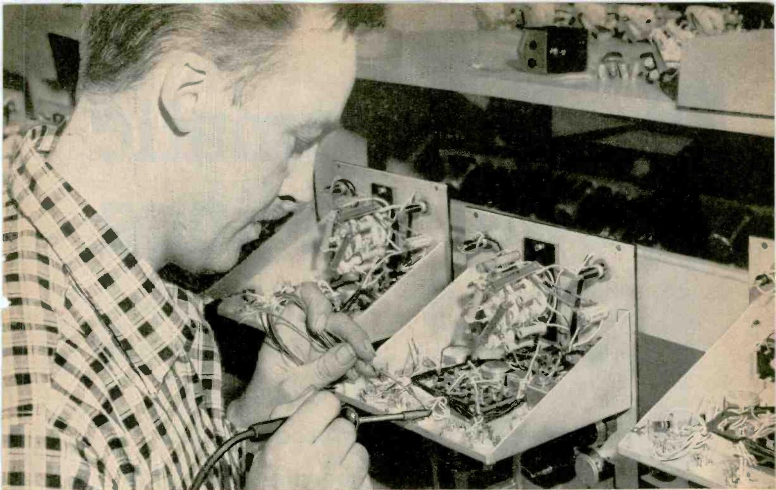
"BEST IRON WE'VE HAD in the plant," says William Fish, a production supervisor of General Radio, Cambridge, Mass. This company has switched to G-E Midget irons for soldering both
