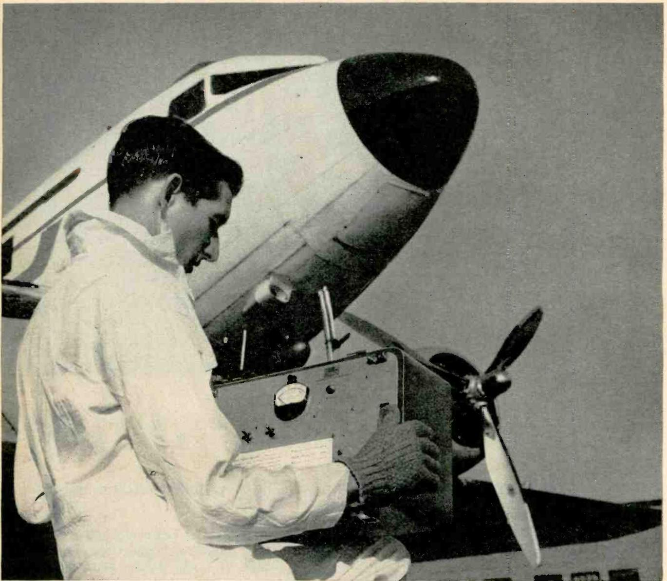
Panel light indicates when radar's ring time exceeds predetermined standard. Other checks can be obtained with frequency indicator and relative power meter.
