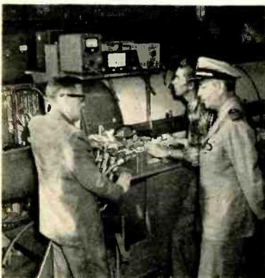
First photo of Polaris hardware shows Polaris test missile's telemetering unit getting check out before being sent to Lockheed's test facility at Cape Canaveral for firing
