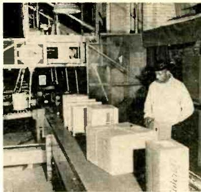
Electronic memory unit (left) activates paddle system (right) to unload conveyor belt as railroaders . . .
