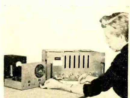
Technician makes proper adjustments of time-interval clock using counter
