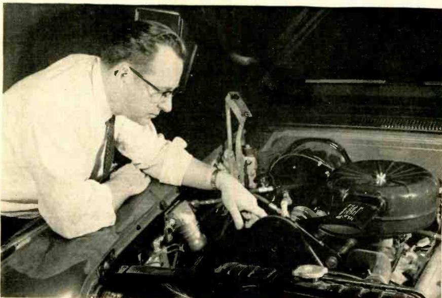
Servo system tied in with power steering on test car is checked by J. Bidwell, department head on GM's research staff. Car follows buried cable carrying low-frequency a-c
