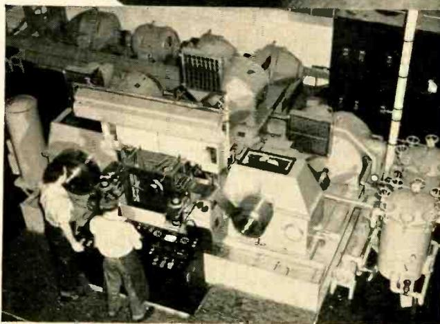
A Sendzimec Mill at General Plate rolls Zirconium foil to 0.00075 inch
