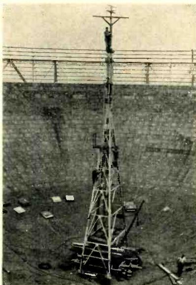
Antenna tower diameter diminishes greatly as its elevation above the reflector increases. This is done to avoid obscuring and scattering radiation from the primary feed. Special structural design is used to prevent the tower from bending when bowl is elevated
