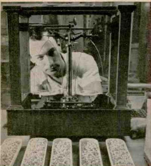
**CERAMIC TUBES MEAN GENERAL ELECTRIC!** A G-E technician is weighing the ceramic spacers of the 7077 triode before firing, to check their density—one of a whole series of special methods developed by General Electric to make practical the use...in tubes...of tough, heat-resistant ceramics.
