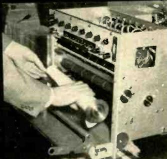
Quick, simple paper loading is done from front; hinged viewing window is removable. About 8" of record visible. All controls on front panel.
