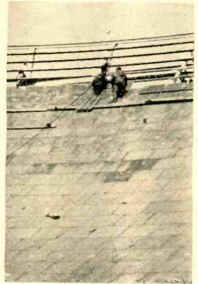
Reflector membrane is built up of 7,000 sheets of 0.5-in. steel plate which are welded to one another and to the support structure. This arrangement gives a high-degree of electrical conductivity, provides adequate pickup of the important 21-centimeter wavelength
