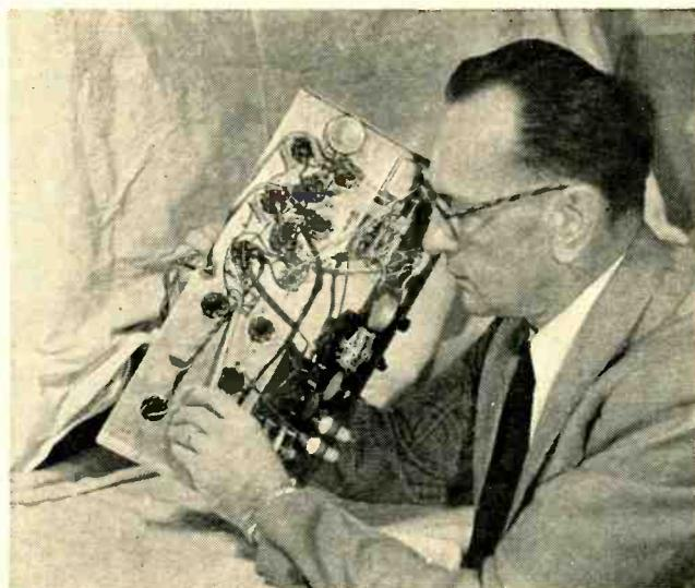
Construction of the differential voltmeter is straightforward. Resistors can be the plain carbon type. Matching is not required because operation is negligibly affected by changes
