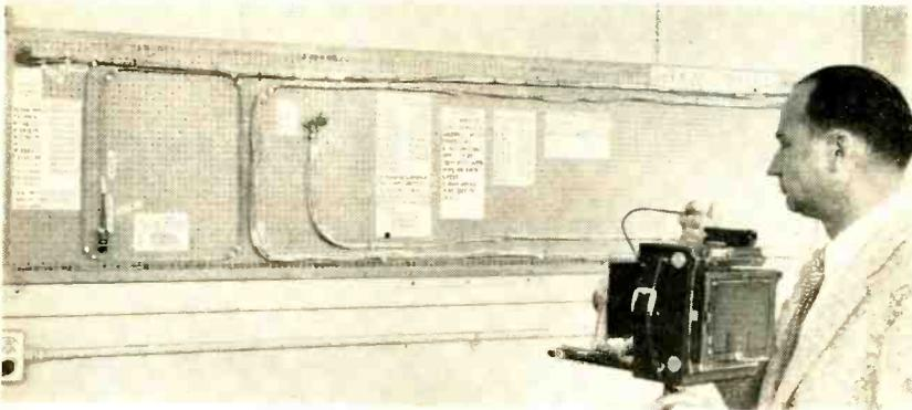
Mockup of wiring harness and assembly directions are photographed for files and production use
