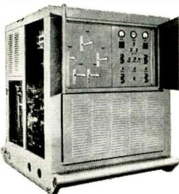
This INET 400-cycle ground power unit was tailor-made for the Atlas. In meeting all of Convair's specifications for pre-flight calibration of electrical systems, the unit operates in parallel with the missile's power system and provides remote control regulation. Frequency regulation is  $\pm 0.2\%$ . With shock load equal to a third of rated output, frequency recovers to  $\pm 0.2\%$  in 0.15 seconds. Voltage regulation is  $\pm 0.5\%$  with recovery time at 0.30 seconds.
