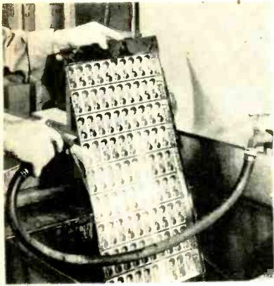
Sheet of name plates is rinsed after unexposed areas are etched off
