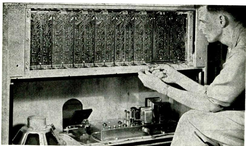
THE FRONT COVER—Engineer installs removable printed-circuit modules in electronic organ. Modules include tone generators, voicing panel and amplifier
