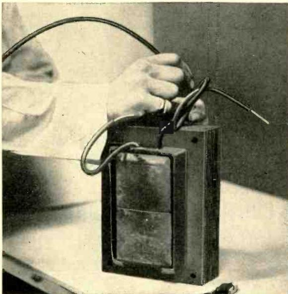
Natvar Isolastane Fibreglas base tubing ▲ and bias tape ▼ fit snugly when applied, and retain their elasticity at continuous operating temperatures up to 155°C. They withstand higher temperatures during manufacturing processes without embrittlement.
