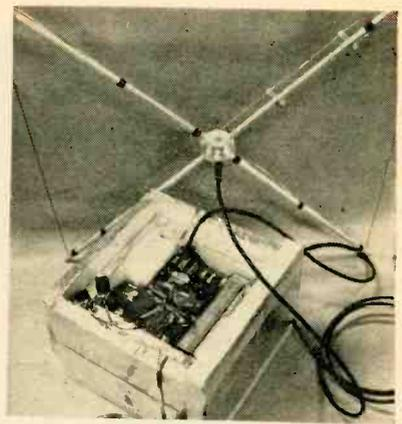
Telemetering equipment operating at 95-mc packaged for flight
