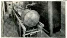
For outstanding vacuum properties, key parts of the Mark 1-T4 accelerator are made of Electronic Grade "A" Nickel. Built by Applied Radiation Corp., Walnut Creek, Cal.
