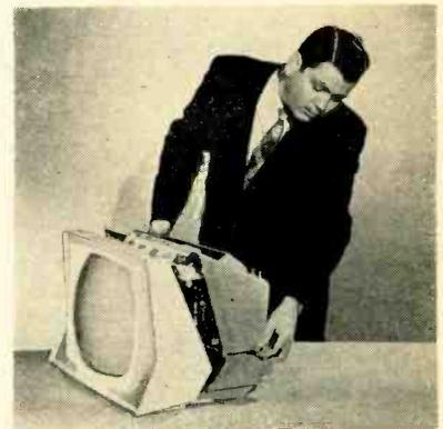
Design engineer shows modular chassis separation used in latest Sylvania portable
