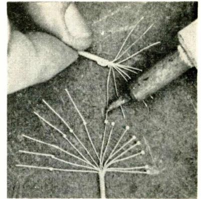
Soldering iron is held about 1/4 in. from dice and heat is conducted down lead
