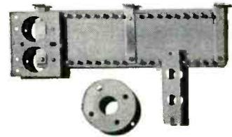
**PRECISE MACHINING AND FABRICATION** are standard benefits of Dilecto laminated plastics. These silicone glass-base parts (coil mountings, aircraft terminal board) were sawed, drilled, punched, and milled in production quantities by C-D-F and customer.
