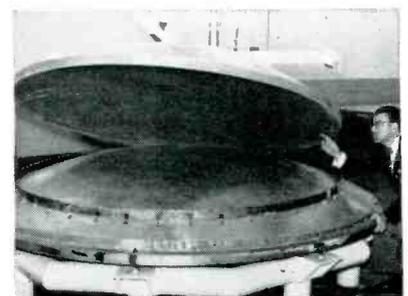
After curing, assembly is lifted off paraboloid face mold
