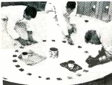
Mounting nut plates and protective caps are fitted to rear structure
