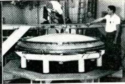
Reflective surface is flame-sprayed on painted face mold
