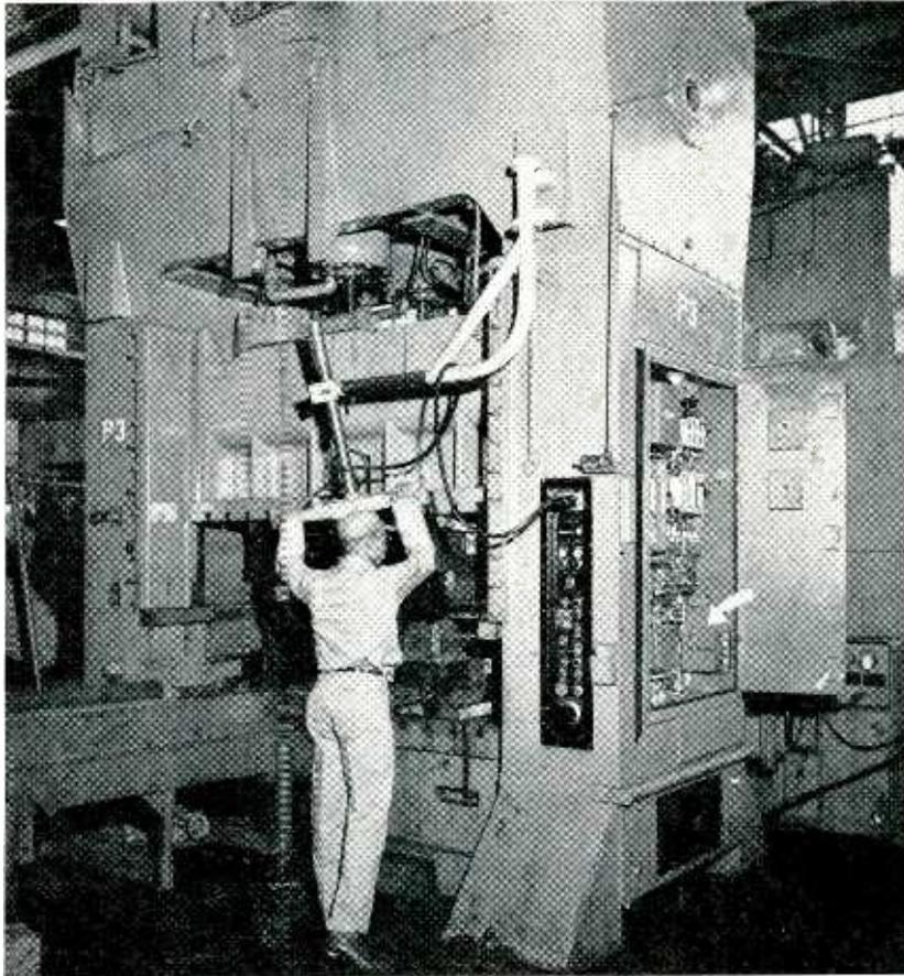
Operator, who is standing before the work, makes an adjustment before starting a cycle. Doors at the right are open to show the power, latch, hold and supply units, which are in the lower right-hand corner of the enclosure (see arrow)
