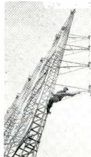
Antennas on this new 96-ft tower at Army Combat Development Experimentation Center's re-transmission station, Fort Ord, Calif., will handle radiophone communications from 300 portable units over 30 channels
