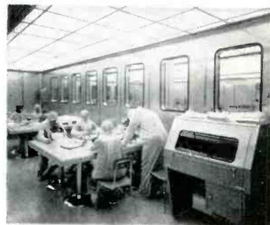
Concentration of airborne contaminants can be held to a few hundred particles (mostly submicron in size) per liter in a room like this
