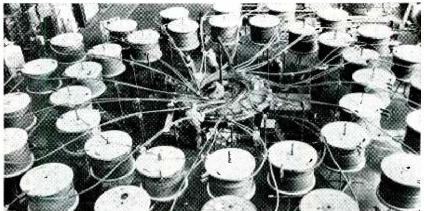
Induction coil being wound (center) is part of electrical power supply system built by GE for driving air through Army's Tullahoma wind tunnel at speeds of Mach 20. Finished copper coil will contain about six miles of cable, weigh 60 tons, stand five ft high, and take one million amps of current
