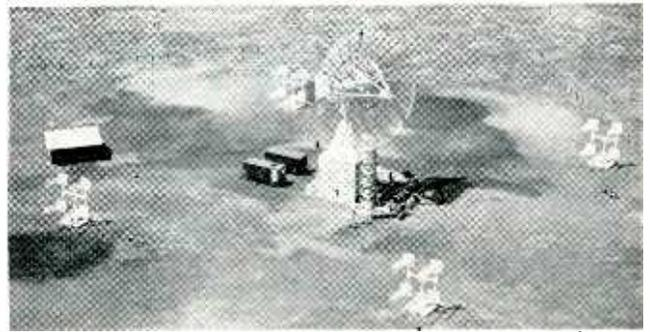
FIG. 3—Aerial photograph of the Hawaii tracking station showing the parabolic receiving antenna and the multiple helix arrays arranged as an interferometer system
