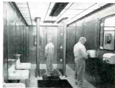
Air shower room of prefabricated clean room installed in Sperry-Farragut plant by Baker. Liquid soap and hot air driers also avoid dust
