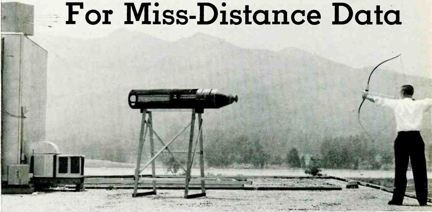
Old-fashioned ballistic missile (arrow) is used to check a new miss-distance indicator. The mdi can detect objects at closing speeds up to Mach 10 and at altitudes to 100,000 feet
