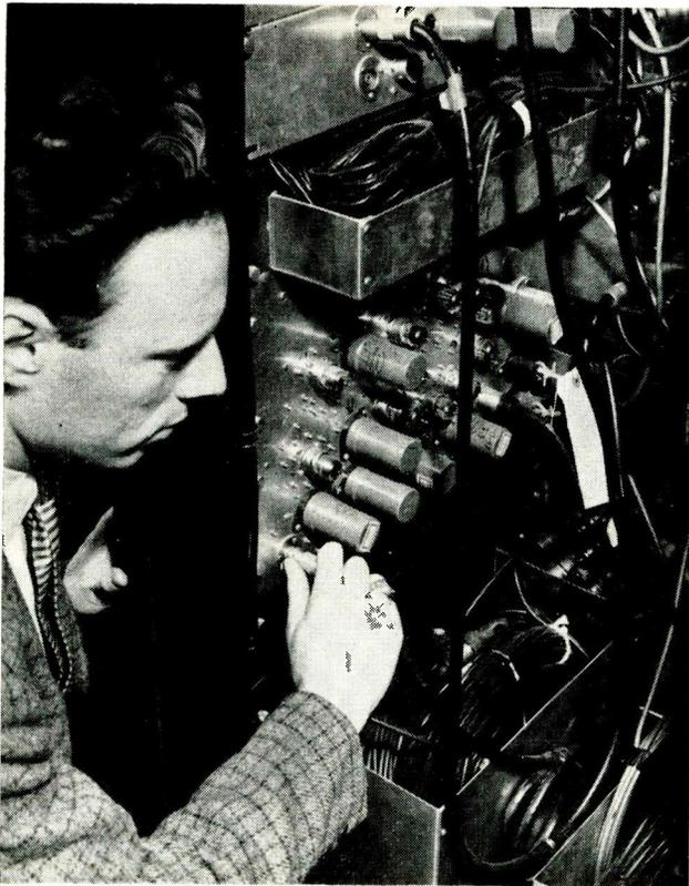
Coaxial cable served as distributed-parameter delay in this experimental 50-mc adder, an early IBM approach to microwave computers
