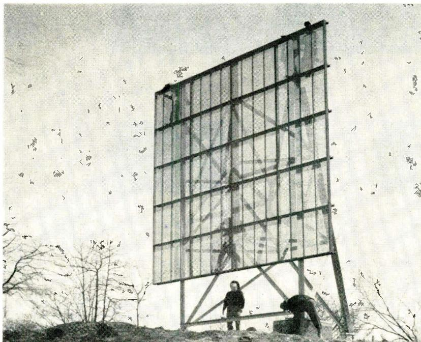
Large passive repeater located on Canton to Philo (Ohio) microwave system of the American Electric Power System
