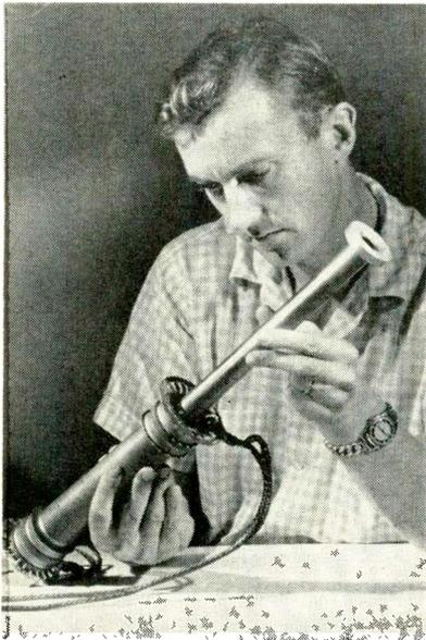
Electron tube in the shape of a hollow cylinder fits like a sleeve over the flame tube attached to a solid-fuel rocket motor. Heat from the burning fuel is converted directly into electricity by the thermionic generator tube which supplies power through wire leads
