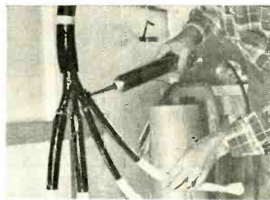
Prepainting with molding compound
