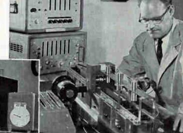
Infrared detectors (vertical cylinders in model) are used in measuring I-beams. Digital computing equipment (behind model) tabulates and notes measurements
