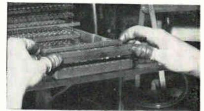
*Operator positions pellet loader over boat, to drop 42 pellets into boat simultaneously*
