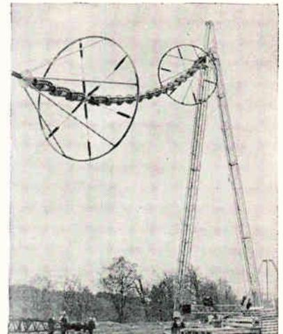
*The U. S. Navy's two-million-watt radio station uses Republic Steel's stainless steel tubing to shield and grade the insulator string to prevent formation of corona and flashover. Top left photo shows welder joining a leg bracket to a section of grading ring. Center photo shows workmen attaching base plate to grading ring at Lapp Insulator's High Voltage Lab in LeRoy, N. Y. Rings and insulators are shown during final testing on dummy tower, right*
