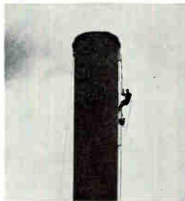
Corrosion check on chimney stack is made by field engineer in bosun's chair. He is using Magnaflux ultrasonic unit
