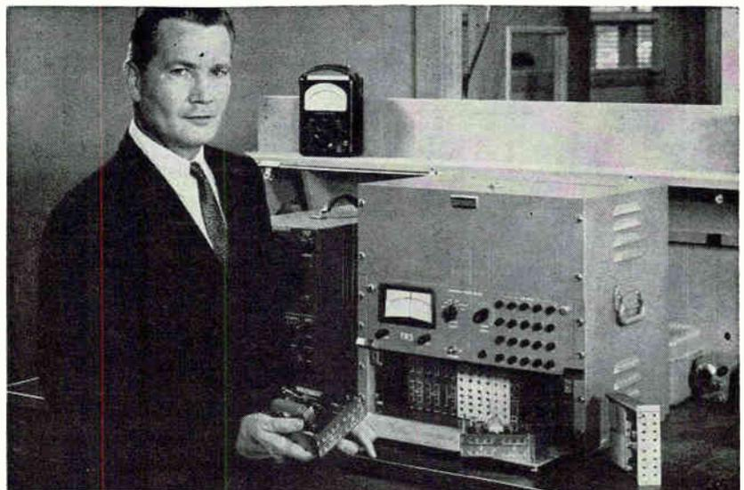
*TR-5 mounting unit built by Electronics Associates makes it possible to assemble special-purpose analog computers using Pace plug-in units*
