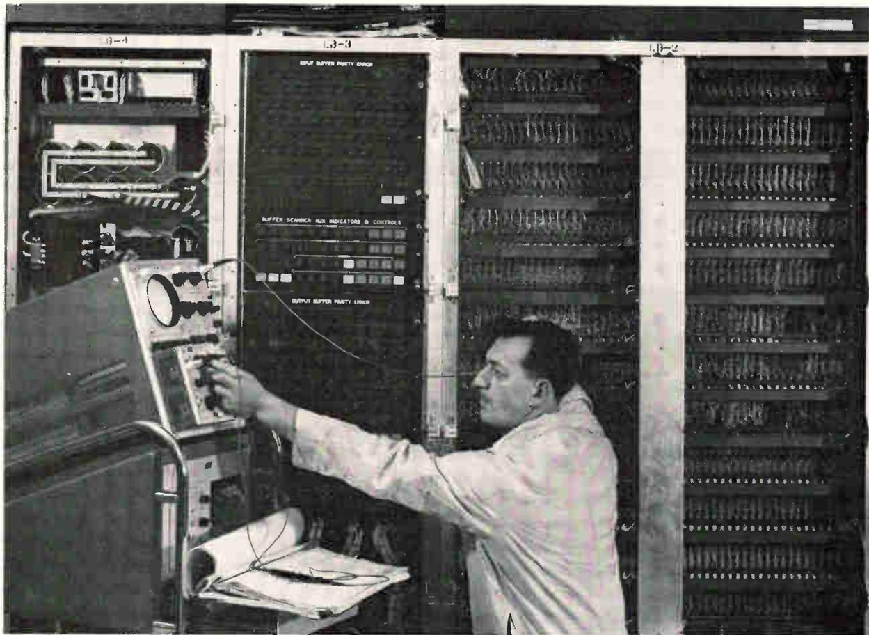
Technician checks the line buffer/scanner unit that provides interface between 100 telegraph lines and CDP. Channel-parity error lights and scanner indicator are housed left of center
