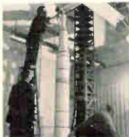
Apollo payload is placed atop a scale model of the Saturn V booster preparatory to wind tunnel tests.
