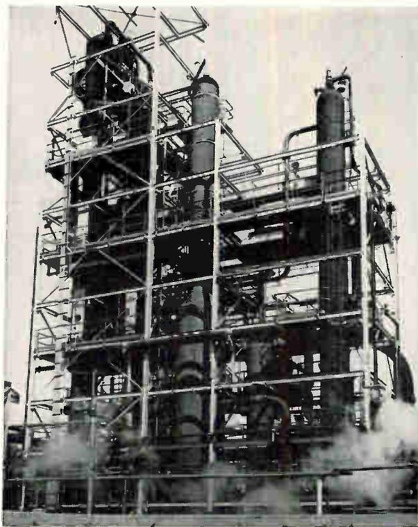
Experimental DDC was tried in Monsanto Chemical's Texas City, Texas, ethylene plant, controlling 10 loops on this distillation column. Savings for a similar 200 loop system were estimated at 500 to 1,000 dollars per loop less than for conventionally equipped loops
