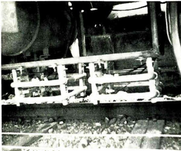
**Upgrading.** JNR is seeking to improve the close-coupled inductive radio system that works off two parallel wires laid between the rails and train-mounted loop coils.
