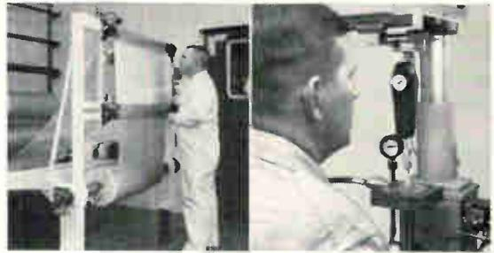
100% of all B-stage—in both rolls and sheet form—is visually inspected at Norplex to insure reliable, inclusion-free bonding sheets.
