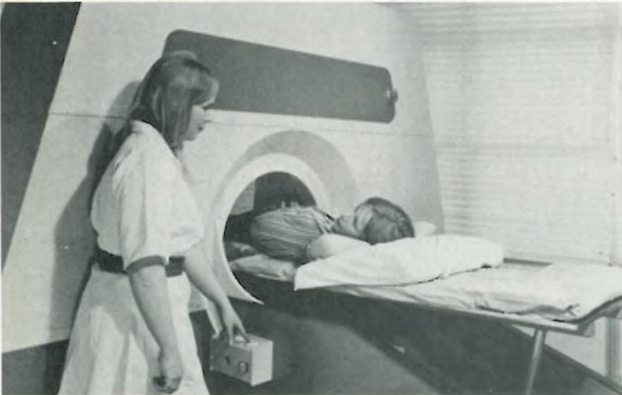
**In operation.** Adjustable couch of EMI's CT 5000 body scanner can be moved through the circular aperture until the section of the body to be examined is directly in line with the X-ray source. The couch of the \$550,000 machine can also be tilted for various angles away from the vertical.
