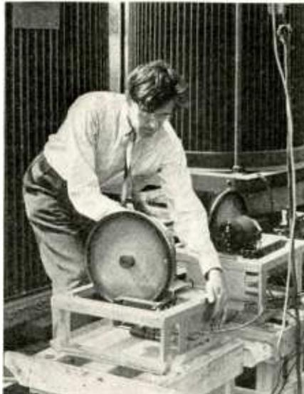
G. D. McCann sets into trial operation one of the fifty fulchronograph surge recorders which have been installed to study lightning. The fulchronograph makes a record of current in a natural lightning stroke throughout its entire duration
