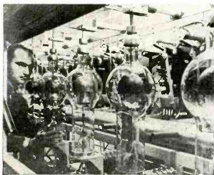
The new 50-kw transmitter of KDKA, at Allison Park, Pa. includes among its many features, an automatic relay shift which banishes interruptions of broadcasts due to rectifier tube failures. In the foreground, above, are rectifier tubes which are cut into the circuit, as required, by automatic tube changing relays shown in the background. Manual changing of tubes is thereby eliminated.
