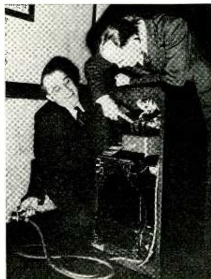
Natural gas drives an electric generator to power the radio receiver shown above. This experimental unit, sponsored by H. Carl Wolf, Natural Gas Company executive, has not yet been developed to a point of practical use in the home
