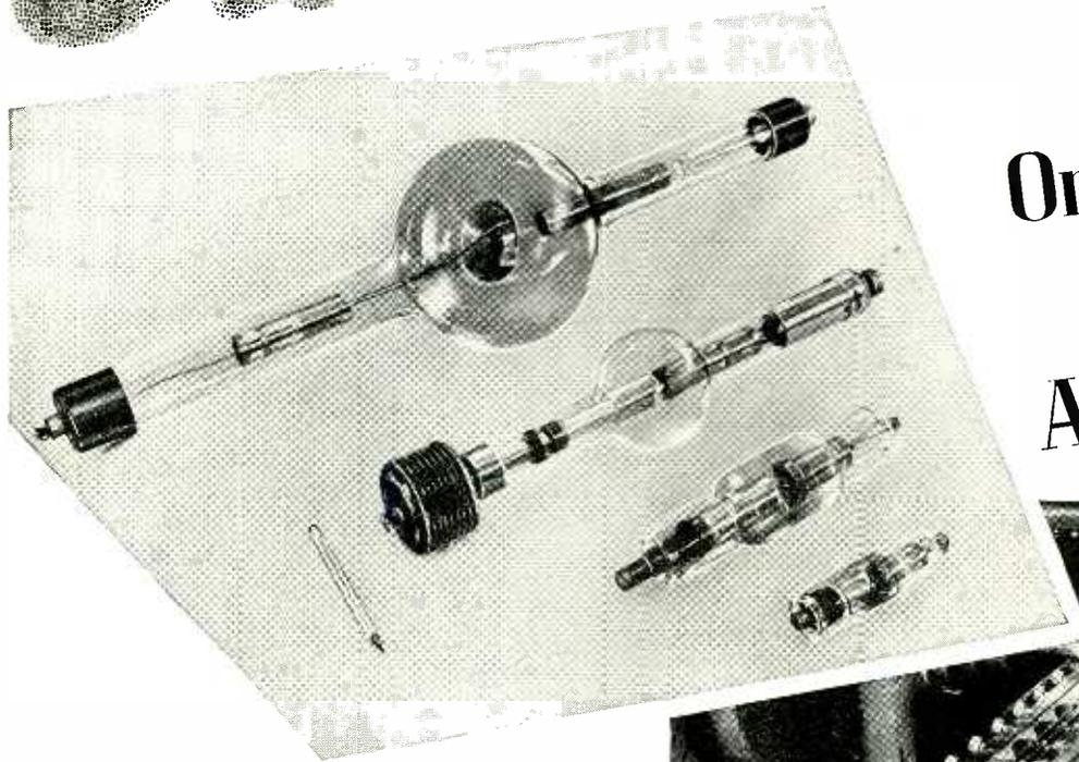
Representative types of X-ray tubes produced by Machlett Laboratories, Inc., Springdale, Conn. At right is shown machining of cathode heads...which must be accurate to 0.0001 of an inch.
