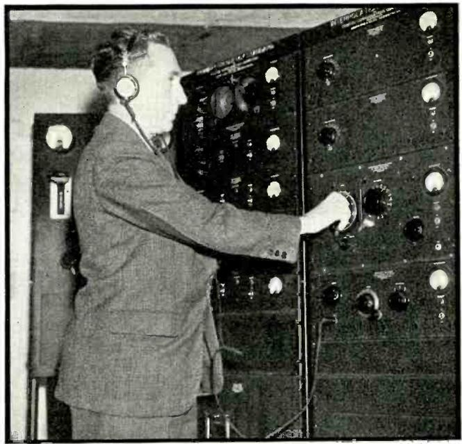
A frequency standard, here operated by Inspector James H. Chapple, is available for checking frequencies throughout the spectrum on which stations are allocated. Harmonics and subharmonics are used to obtain off-crystal frequencies
