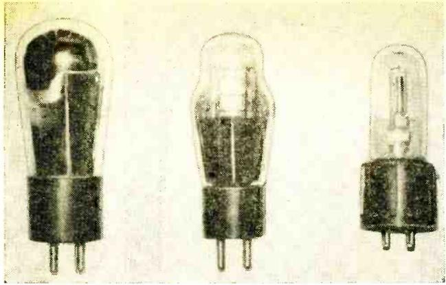
was held in position by the side wiping contacts. In place of the bayonet pin (which not only held the UV tubes in the sockets, but also provided orientation of the tube pins to the proper contacts) UX sockets used two large pins for the filament leads. Thus, the tube would only fit into the UX sockets when the large filament pins were inserted into the proper socket holes. Usually, broadcast receivers made *prior* to 1925 were equipped with UV sockets while those made later had UX sockets.
