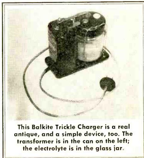
This Balkite Trickle Charger is a real antique, and a simple device, too. The transformer is in the can on the left; the electrolyte is in the glass jar.
