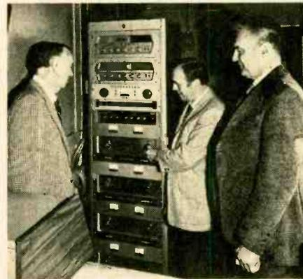
This shot of the audio control room at Notre Dame Stadium shows the four Crown DC-300A amplifiers, as well as the Spotmaster 5 BEM-2005 audio console and Crown VFX-2 filter.
