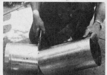
Fig. 9. The damper assembly is generally long enough to pass through thin-walled buildings. If you need extra length, standard 8-in. flue pipe obtainable at local plumbing outlets can be cut to size.
