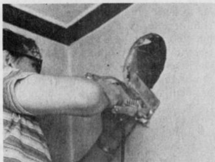
Fig. 4. If you have made a measuring error and find a stud running past the hole, don't panic. The wall will stand even if you cut through one stud. Use a saber saw to trim the stud so the cuts correspond to the circular duct pattern.
