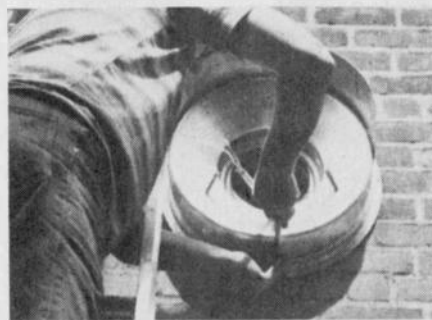
Fig. 10. If you have no one to help when mounting the fan assembly, cut down the overall weight by removing the motor and fan from the rain shield. Secure the shield to the wall and then install the motor and fan. Note the electric wires from inside the house coming up through the shield.
