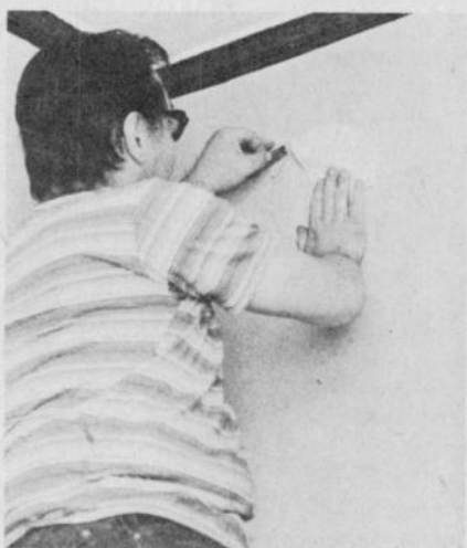
Fig. 1. Pick a location for the grille-damper, and make certain it's between two wall studs. Using the duct as a template, scribe the outline on the wall and then use a razor to cut away the wallpaper.
