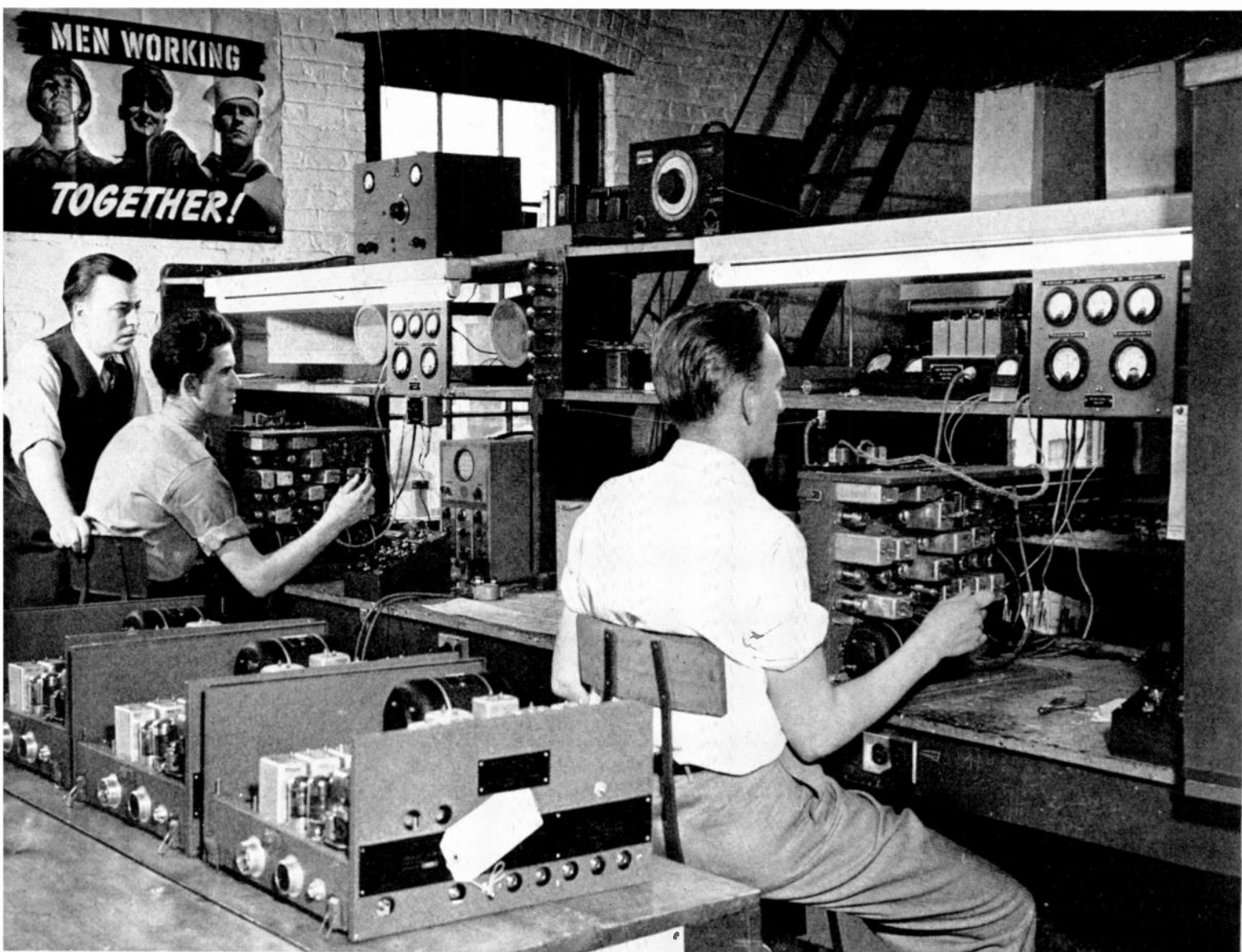
FIG. 6, RIGHT, 1ST POSITION AND, LEFT, 2ND POSITION OF FINAL TEST, WHERE CIRCUITS ARE CHECKED AND CONDENSERS ARE ALIGNED
