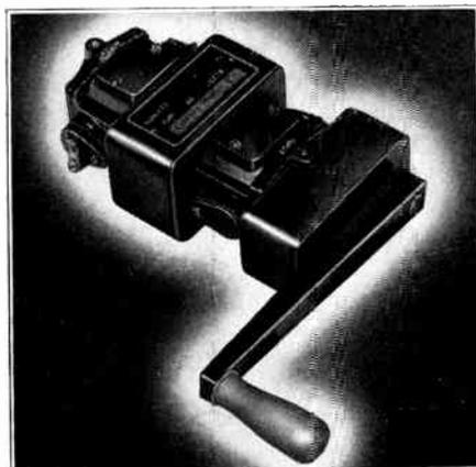
14 FIG. 3. 6-LB. GENERATOR DELIVERS 30 WATTS
