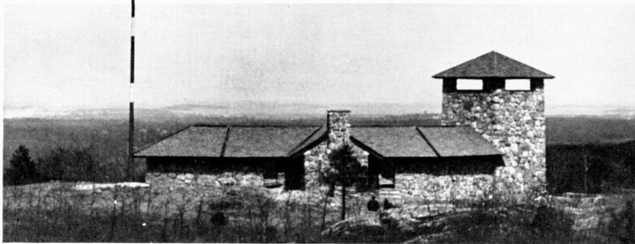
FIG. 6. MAIN STATION OF METROPOLITAN DISTRICT COMMISSION IS ON HIGH GROUND OVERLOOKING BOSTON HARBOR
