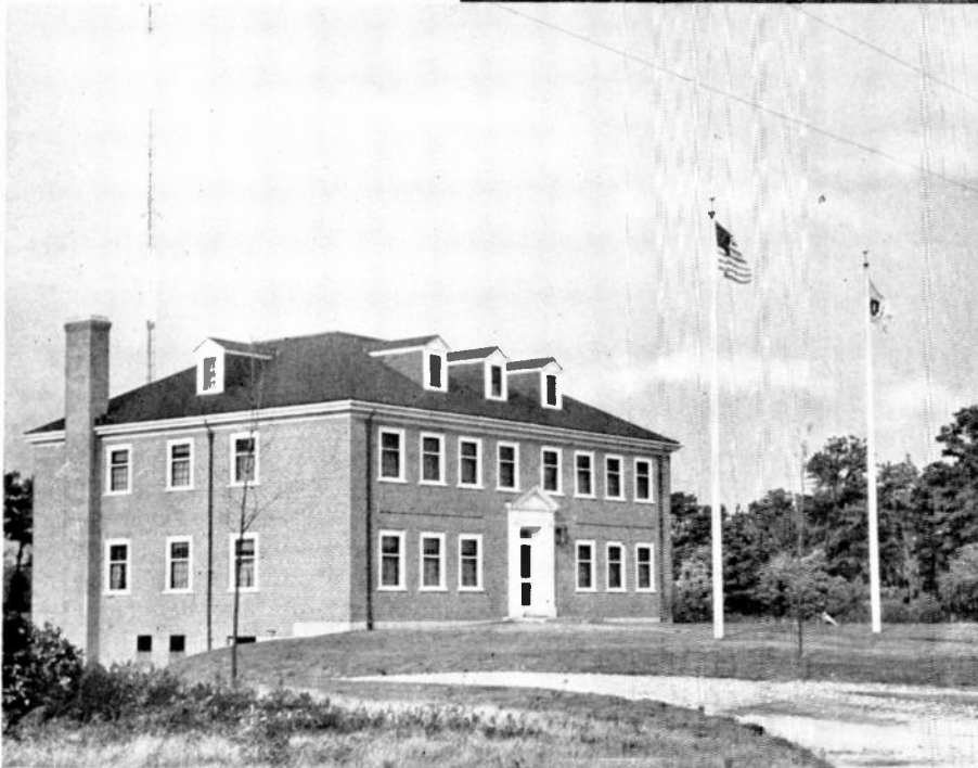
FIG. 3, BELOW. A TYPICAL SUBSTATION OF THE MASSACHUSETTS STATE POLICE, AT YARMOUTH. AT THE LEFT CAN BE SEEN THE GUYED WINCHARGER TYPE OF ANTENNA MAST
