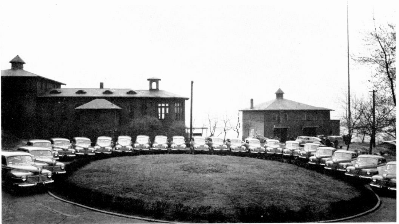
FIG. 2. SOME OF THE PITTSBURGH POLICE PATROL CARS LINED UP FOR INSPECTION AFTER THE INSTALLATION OF 2-WAY FM EQUIPMENT. THEY PROVIDE COMPLETE COVERAGE NOW, EVEN WHERE AM COULD NOT REACH
