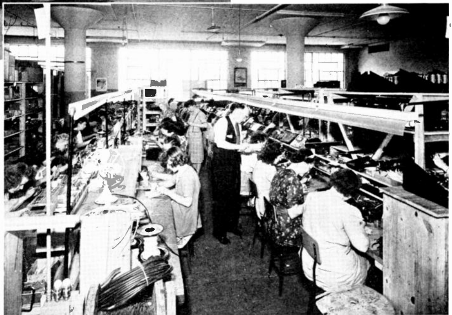
APPARATUS ASSEMBLY AT THE CHICAGO PLANT. PRESS WIRELESS, INC. ALSO OPERATES FACTORIES AT HICKSVILLE, N. Y. AND AT MOUNTAIN GROVE, MO.
