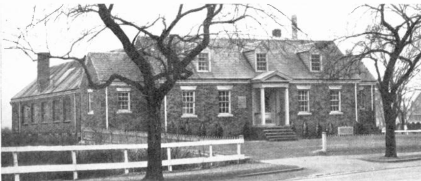
NEW OFFICES AND DEMONSTRATION LABORATORY OF ELECTRICAL APPARATUS COMPANY AT 1200 SOLDIERS FIELD ROAD, BOSTON, ADJACENT TO HARVARD UNIVERSITY
