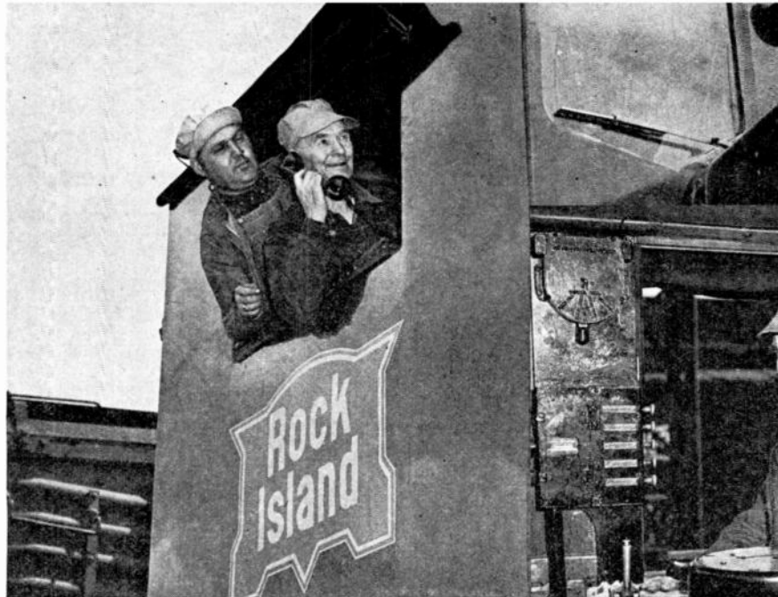
FIRST OF THE ROCK ISLAND'S 2-WAY FM INSTALLATIONS ARE FOR USE BETWEEN DISPATCHER'S OFFICE AND SWITCHING ENGINES. CONVENTIONAL METHOD IS TO SEND COURIERS ON FOOT TO DELIVER MESSAGES TO THE ENGINEERS
