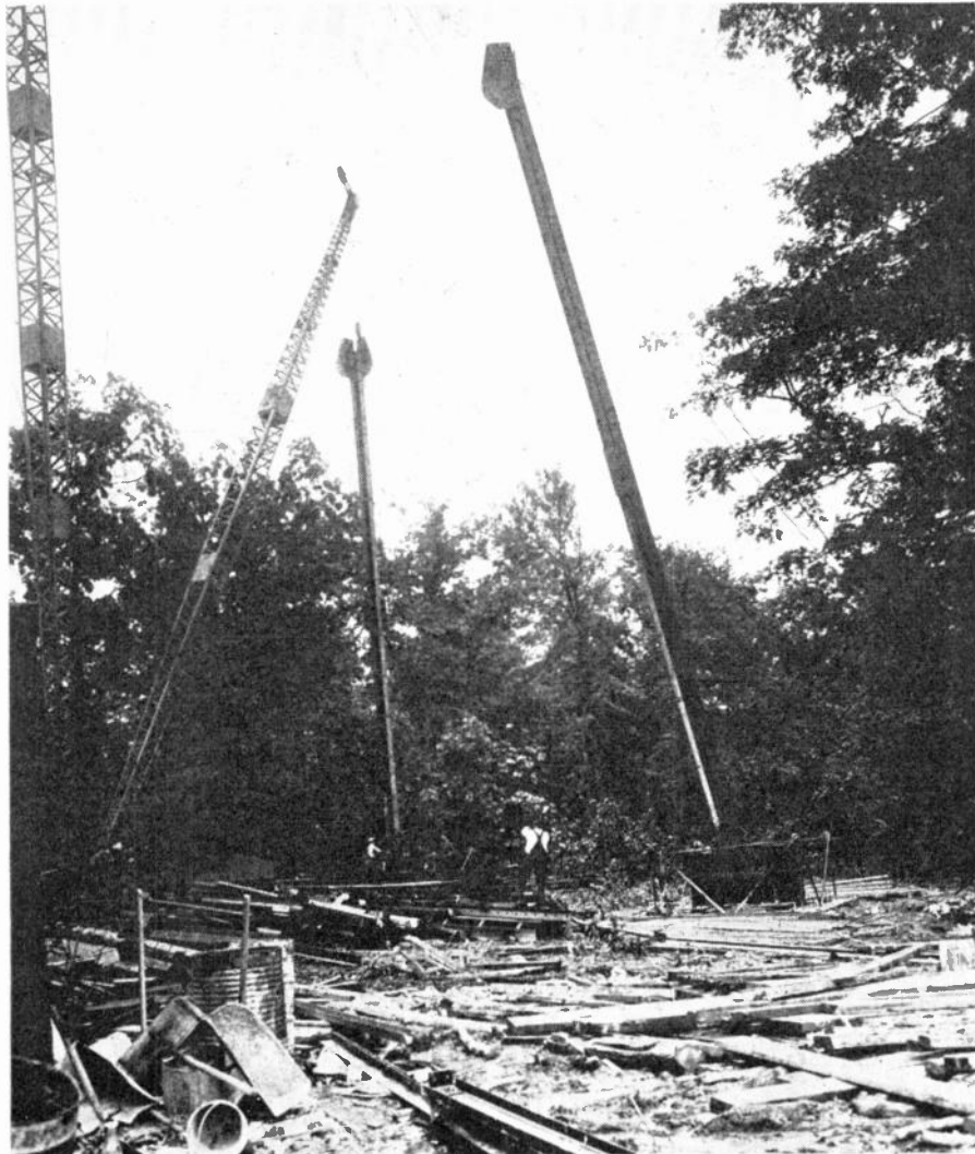
CONSTRUCTION OF THE ALPINE STATION WAS STARTED EARLY IN 1937
