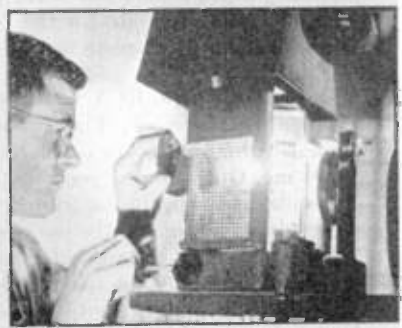
METALLURGY — Spectrographic Analysis of the Rare Metals Used in Vacuum Tubes
