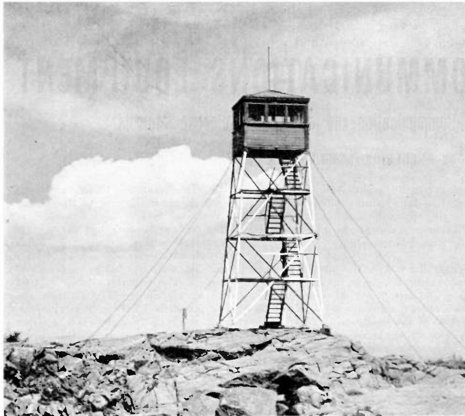
FIG. 13. CAR SIGNALS ARE PICKED UP HERE ON MT. KEARSARGE AND ARE THEN BEAMED BY FM RELAY TO CONCORD HEADQUARTERS, 28 MILES DISTANT
