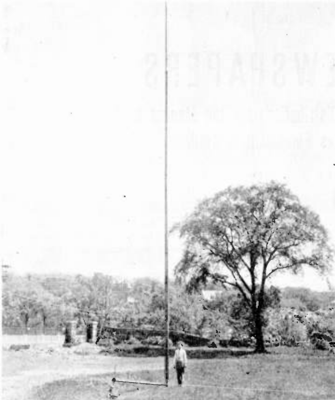
ABOVE, TWO MEN CAN ERECT THIS 75-FT. MAST WITHOUT SPECIAL EQUIPMENT. RIGHT, THIS IS AN IDEAL MAST FOR USE ON APARTMENT HOUSE ROOFS
