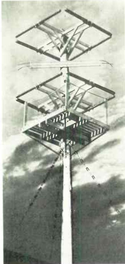
FIG. 35. TELEVISION SOUND TRANSMITTING ANTENNA AT MAIN STATION
