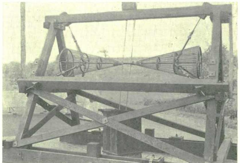
FIG. 32. CONICAL DOUBLET USED AS THE PICTURE TRANSMITTING ANTENNA
