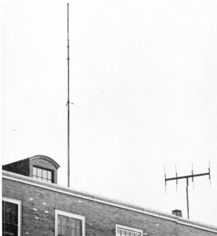
PENDING ERECTION OF NEW TURNSTILE, WBKY IS GETTING EXCELLENT RESULTS WITH POLICE TYPE COAXIAL ANTENNA
